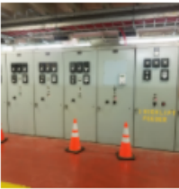
Representative Switchgear to be Replaced under CIP 111001
