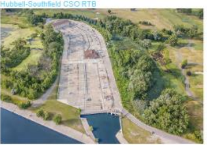
Figure 41. Hubbell-Southfield CSO RTB The Hubbell-Southfield CSO RTB is one of GLWA's most active, longest operating CSO facilities and the largest on the Rouge River. Since August 1999, it has been effectively capturing and treating combined sewage through screening, settling and disinfection to meet discharge permit requirements that protect public health. Sized to fit into the available land and site constraints, the basin has a 22-million-gallon storage capacity. Located next to the Tournament Players Championship Golf Course (TPC) in Dearborn, this RTB serves as an example of how these facilities can be good neighbors and blend in with the surrounding environment. The facility features an innovative design component that enables three different operational modes within the RTB and prevents resuspension of solids during large storms with high flow rates.
