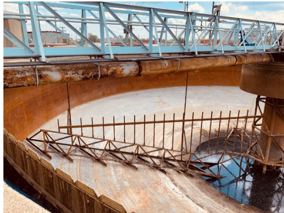
Newly repaired No. 2 Thickener
