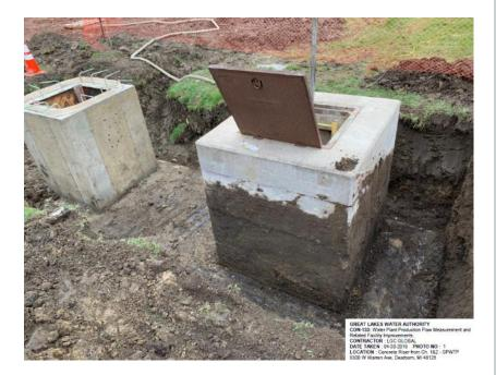
Water proofing concrete risers for metering chamber
