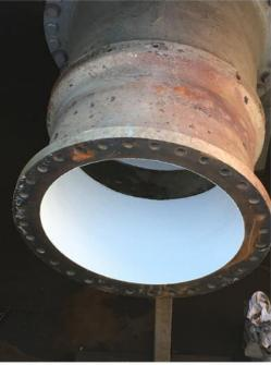
Phota 3: Second coat of paint applied at the divergent section of VM-6 at the NEWTP.
