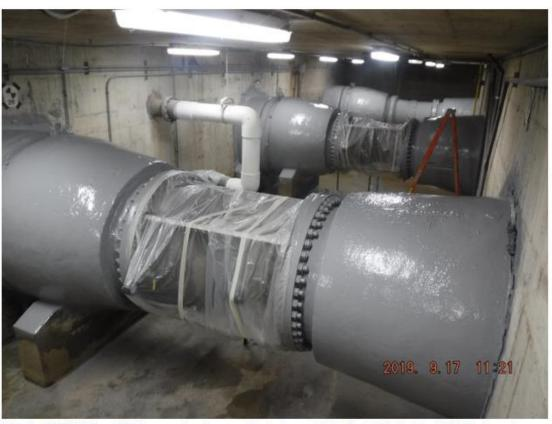
Photo 3: VM-2, VM-1, and VM-3, as seen from foreground to background, in the Venturi Vault at the SWWTP facing east.
