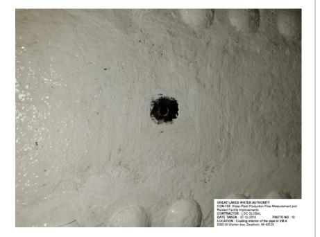
*Rehabbed pressure port for venturi meter*
