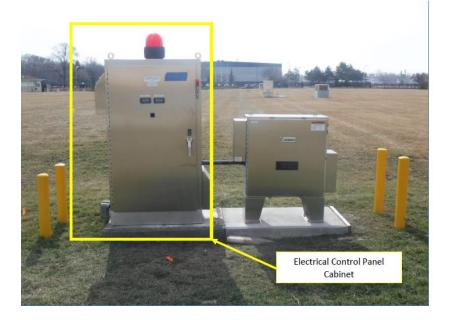
*Typical new VM-6 Flood float/switch and sum pumps system.*
