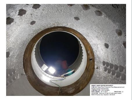
Super metal applied to joint in metering chamber
