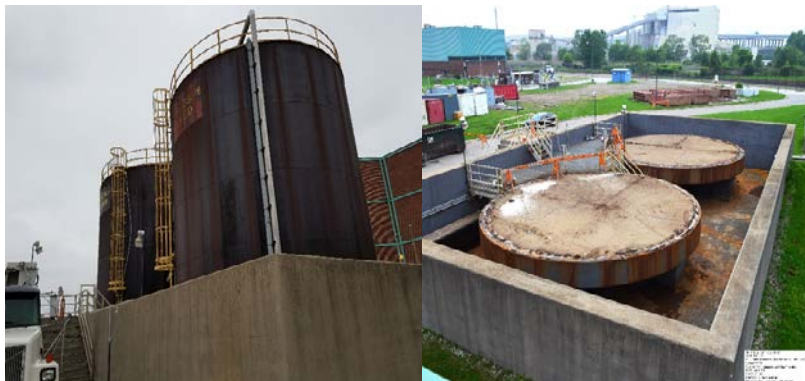
Before and after demolition of 24 years old Ferric Chloride storage tanks
