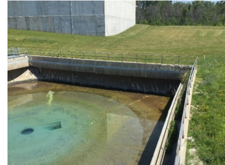
Raw sludge clarifier at Lake Huron WTP
