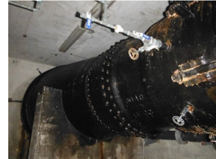
Water production flow metering device
