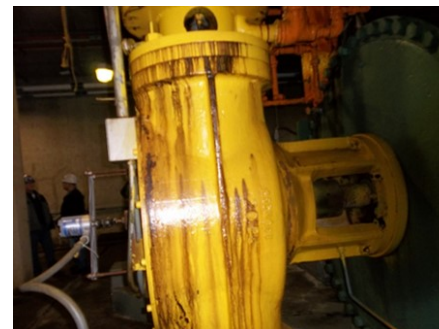
Oil hydraulic valve actuators leaking oil
