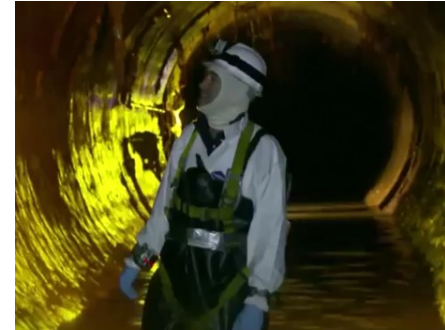
Visual inspection of a large sewer
