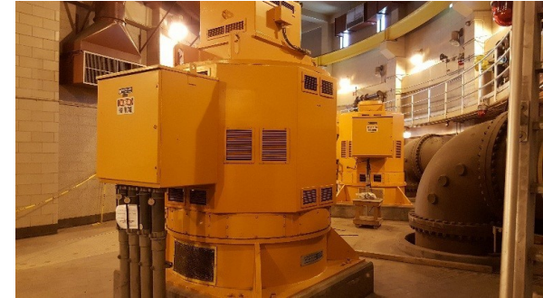
Main Raw Sewage Pumps at Pump Station 2
