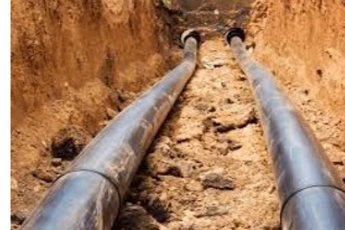
Water main installation
