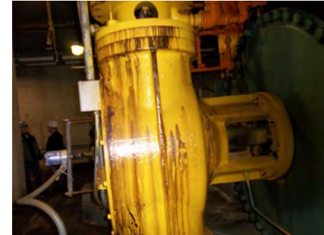
Oil hydraulic valve actuators leaking oil
