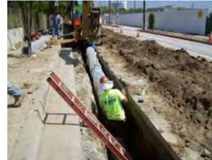
Water main being replaced
