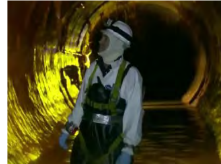
Example inspection of a large sewer
