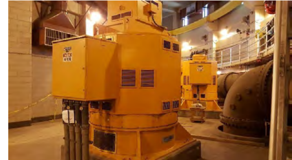
Main Raw Sewage Pumps at Pump Station 2
