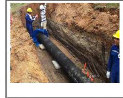
Water main being installed
