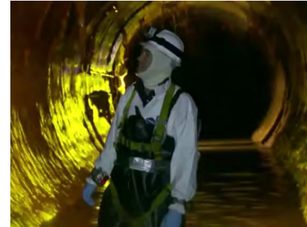
Visual inspection of a large sewer
