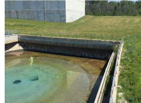
Raw sludge clarifier at Lake Huron WTP
