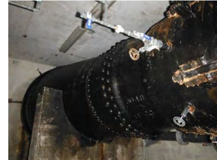
Water production flow metering device
