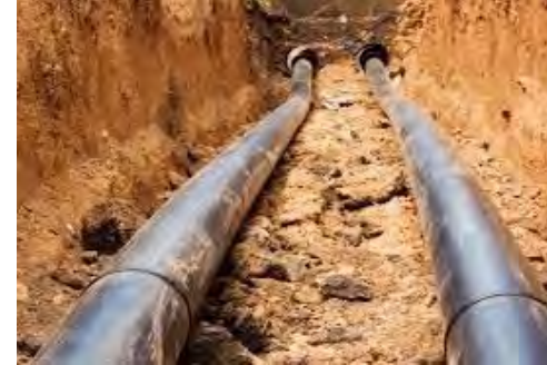
Water main installation
