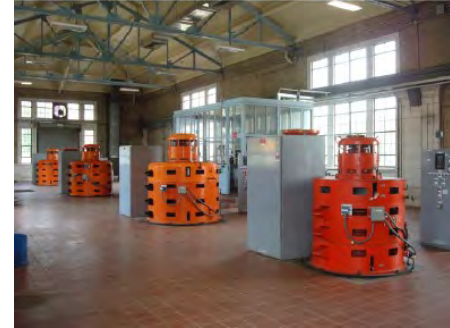
Sanitary pumps at Fairview Pumping Station
