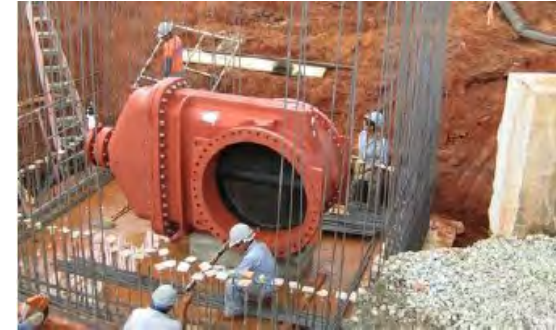
A large valve for a transmission pipe
