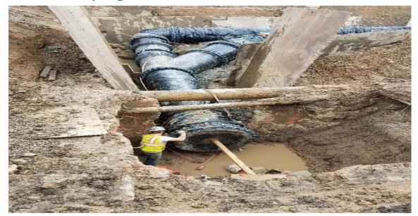
Installation of 42" Blind Flange / Cap
