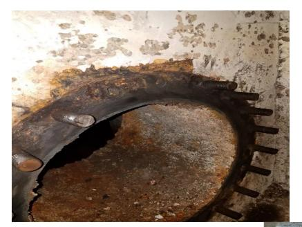
Removed existing 24" Butterfly Valve & Wall Thimble
