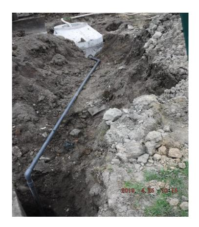
Springwells Plant – Sump discharge piping for de-watering located at Chamber 3-4.
