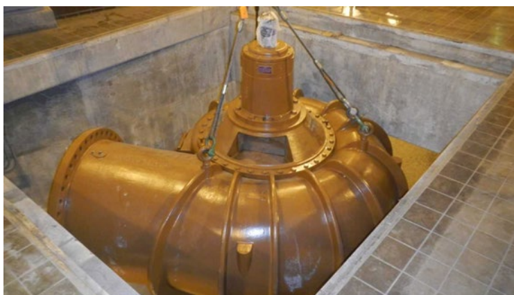
Pump No. 11 installation
