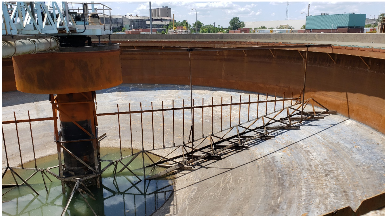
Rehabilitated primary sludge thickener rake/mechanism
