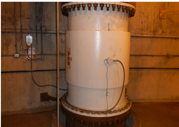
New Flowmeter for Pump No. 11
