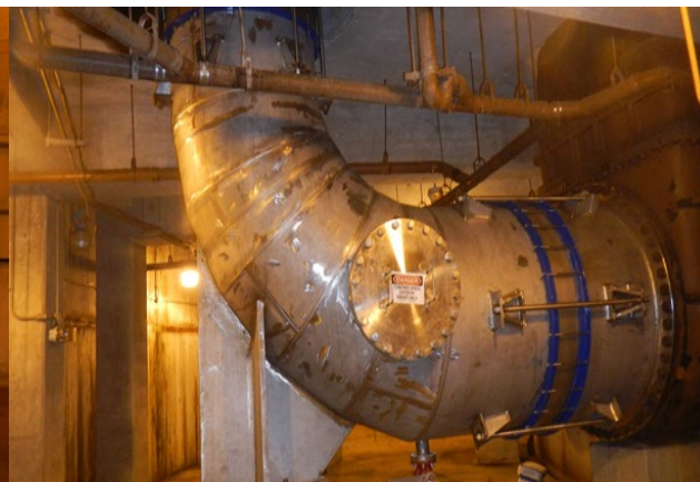
New Suction Elbow for Pump No.
