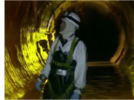
Example inspection of a large sewer
