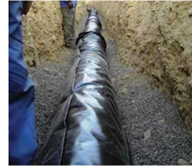
Water main being laid
