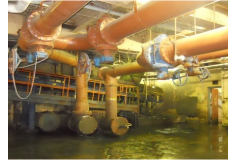
Sludge Feed Pumps
