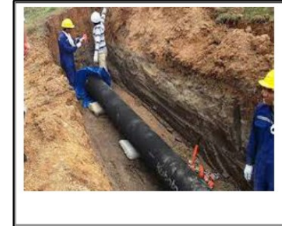
Water main being installed
