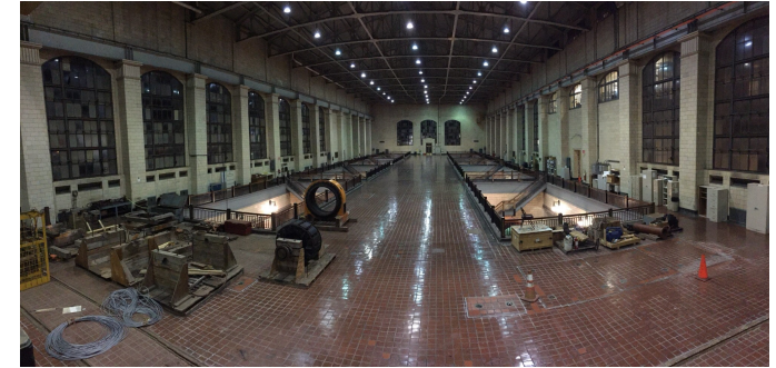
High Lift Station viewed from Low Lift Station operating floor showing high lift pump pits and windows to be replaced.
