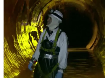
Visual inspection of a large sewer
