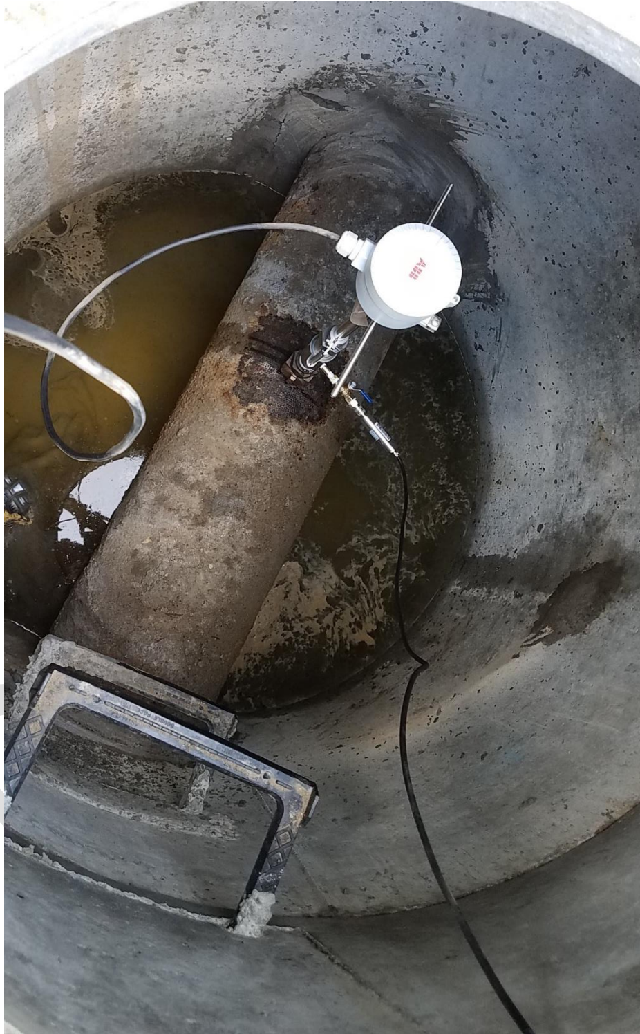
Figure 2-24 Insertion Mag Flow Meter Installation in Dearborn DB1
