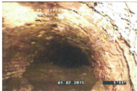
Sewer tap piping in B009 outfall (left) and sludge buildup and poor masonry in B007 outfall (right)
