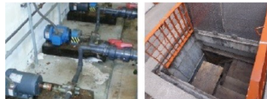
Retrofitted chemical feed pump replacement at Puritan-Fenkell RTB and makeshift wooden stairs to enter Basin Valve Gallery
