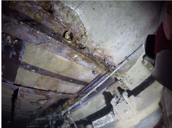
Exposed rebar
