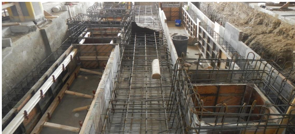
Installation of re-steel and wall forms for the PE flowmeter risers.
