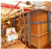
Significant SFE & Secondary Water Pump Station and pipe corrosion, requiring equipment and building rehabilitation. No redundancy for power supply to SFE pump station. Latest cooling oil test (DGA) indicates potential issues with two 5kV Transformers
