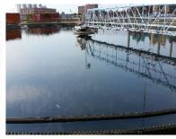
Only one or maximum two out of total 25 secondary clarifiers can be taken out of service at a time for repairs. Secondary system has a lot of moving parts and equipment. A long term (8 years) rehabilitation program for the secondary clarifiers needs to be
