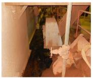
Ash crusher system was last rehabilitated 15 years ago and near the end of its useful life, due to Complex I decommissioning dry ash system needs to be reconfigured and rehabilitated
