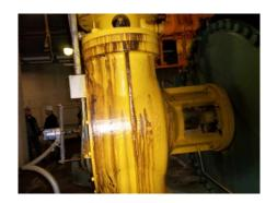
Oil hydraulic valve actuators leaking oil
