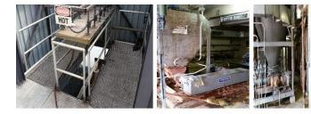
The existing scum system is complicated to operate and difficult to maintain, equipment remains out of service for extended period. The scum beaches need better enclosure and heating system, during extreme cold conditions scum collection system get frozen
