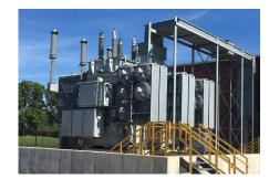
The new 3rd 120/13.8 kV Transformer installed and owned by the Great Lakes Water Authority waiting for the 3rd Primary Electric Feed Line to be installed and energized
