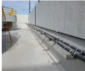
*Heat-Traced Ferric Chloride Piping*
