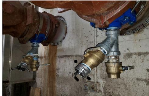
*New 3-inch diameter drain lines installed for the 18-inch diameter Sludge Feed Piping for Sludge Storage Tanks 5 and 6, JOC Task 70.JOC Task J2-01*
