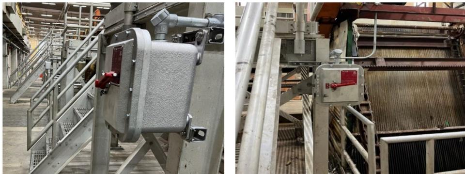
*New local disconnects installed for the bar racks at Pump Station 2*
