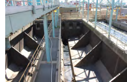
Pump Station 2, Grit channels
