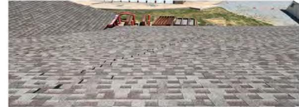
• The previous installation on roof area 2 also failed to follow the required "step-down" installation method. As seen in the picture above, the shingle seams fall >4" from each other. This is a very common mistake found on
