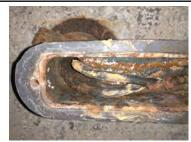
Leaking Conduit in Drain Vault
