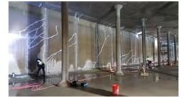
Imlay Booster Station: Sealing interior wall cracks
