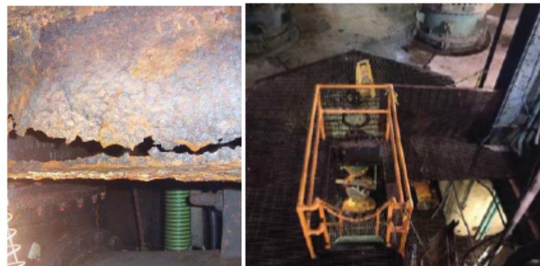
Deteriorated support beams holding up Low Lift Station Dewatering and Sump Pumps at Elev. 42'-0" (left). Deteriorated grating and access ship's ladder in Low Lift Station - Looking down at Elev. 50'-0" and 42'-0" from Elev. 62'-0" (right).
