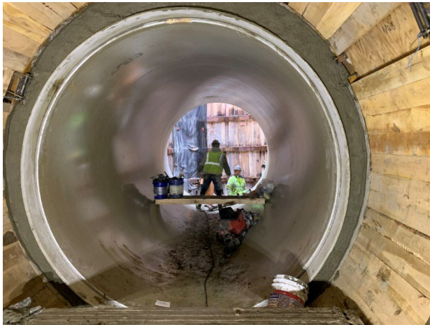
Grand Connection primary liner under construction
