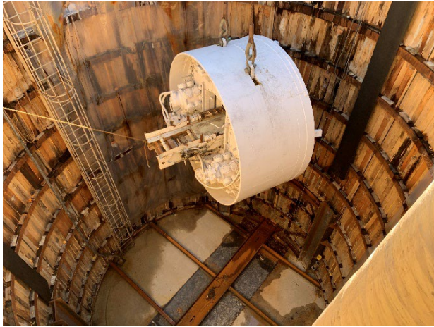
Section of tunnel boring machine being lowered into the launching shaft
