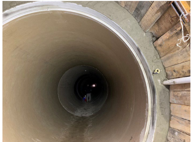
Progress on lining and grouting of Grand Connection
