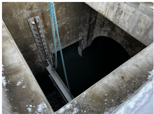
Permanent gate structure under construction at DRI end of Grand Connection
