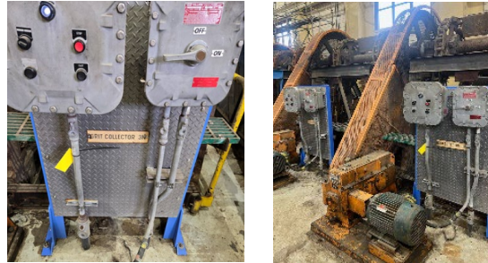
New mounting panels for Grit Collector #3 electrical controls are shown above
