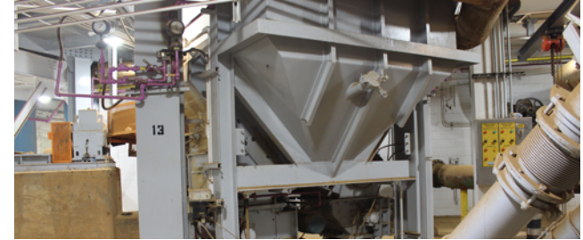
WRRF Rehabilitation of the Ash Handling Systems
