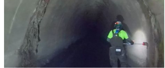
Conveyance System Repairs (Sewers)
