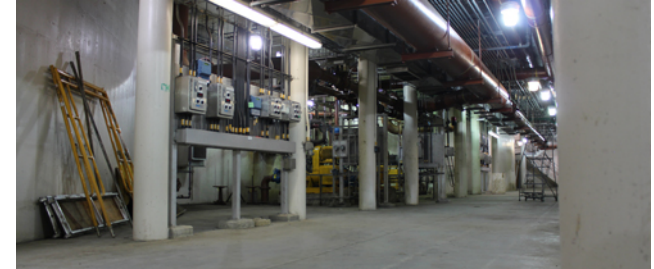
Rehabilitation of Sludge Processing Complexes A and B
