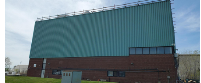
2022 WRRF Roof Improvements Project
