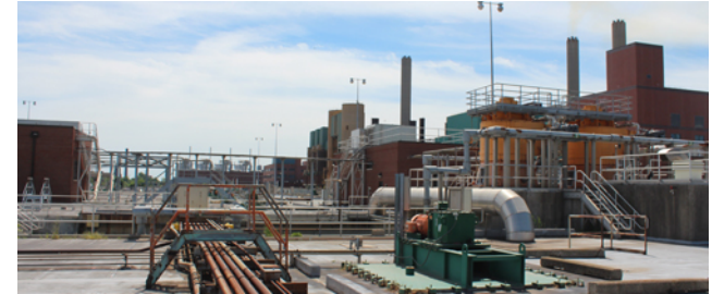
WRRF Aeration Improvements 1 and 2
