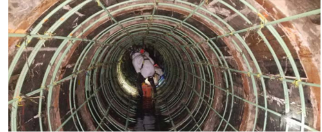
CON-149, Emergency Sewer Repair
