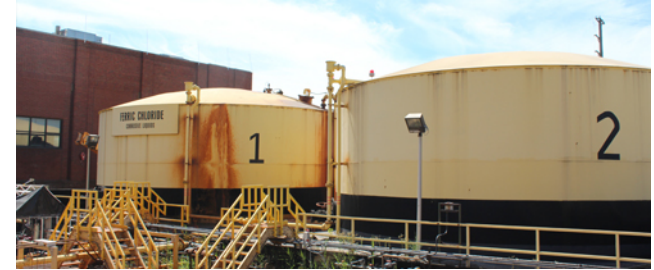
WRRF Rehabilitation of Ferric Chloride Feed System in PS-1 and Complex B Sludge Lines
