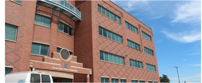
WRRF Facility Optimization Program
