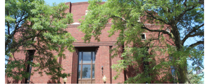
WRRF PS No. 1 Improvements
