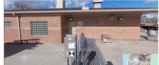
CSO Hubbell Southfield VR-8 Gate Improvements
