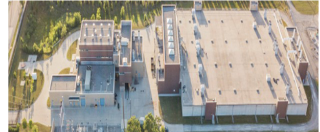
Oakwood and Leib CSO Facilities Improvement Project
