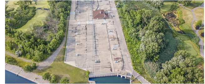
Hubbell Southfield CSO Facility
