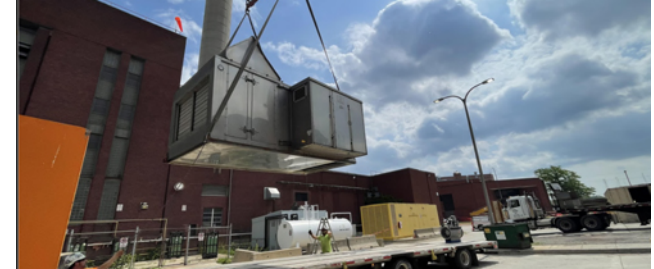
PS 1 Rack and Grit HVAC System Upgrade
