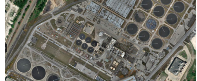
WRRF Roof Improvements - Phase II
