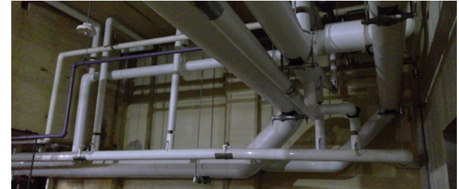
Condensate Return, and Compressed Air Piping
