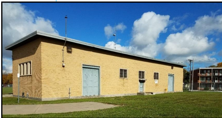
Figure 21. Eastside Pump Station
