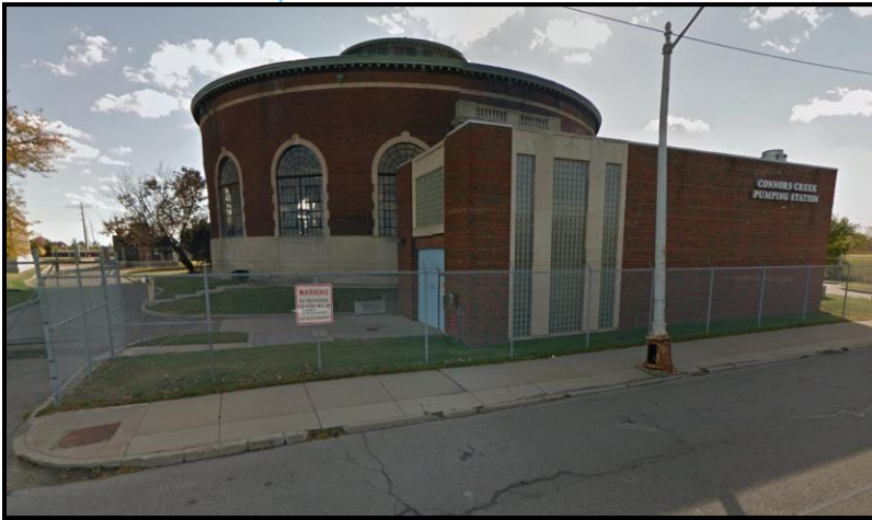
Figure 55. Conner Creek Pump Station
