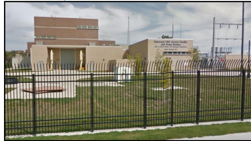
Figure 62. Oakwood Pump Station
