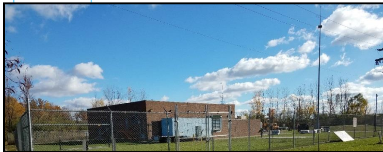
Figure 38. Ypsilanti Pump Station
