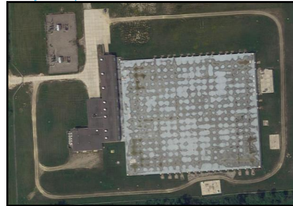
Figure 28. Imlay Pump Station
