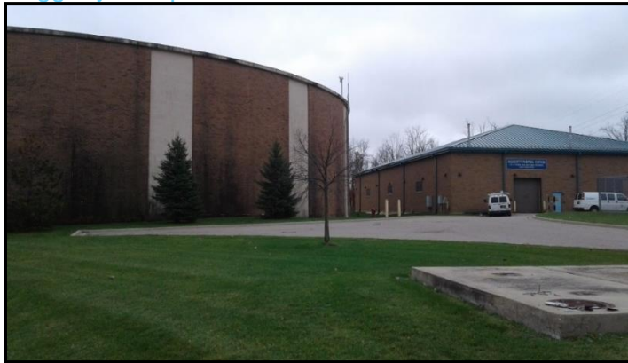
Figure 23. Haggerty Pump Station
