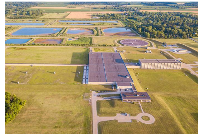
Figure 3. Lake Huron WTP
