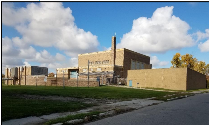
Figure 59. Freud Pump Station
