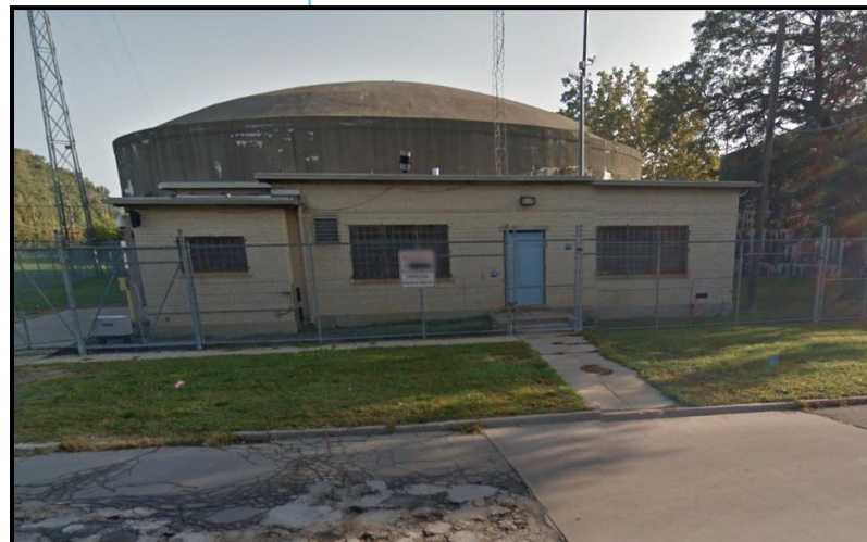
Figure 22. Electric Avenue Pump Station
