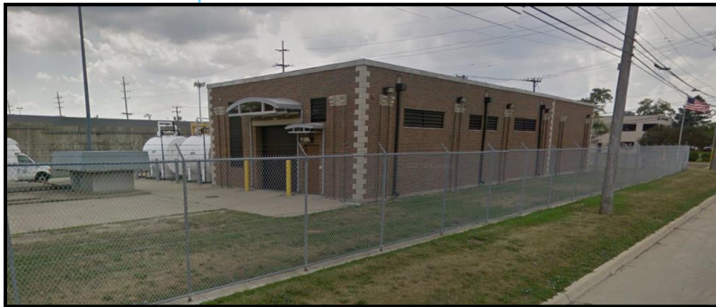
Figure 35. Schoolcraft Pump Station
