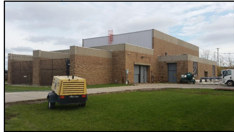
Figure 61. Northeast Pump Station
