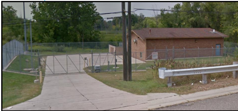
Figure 32. Orion Pump Station
