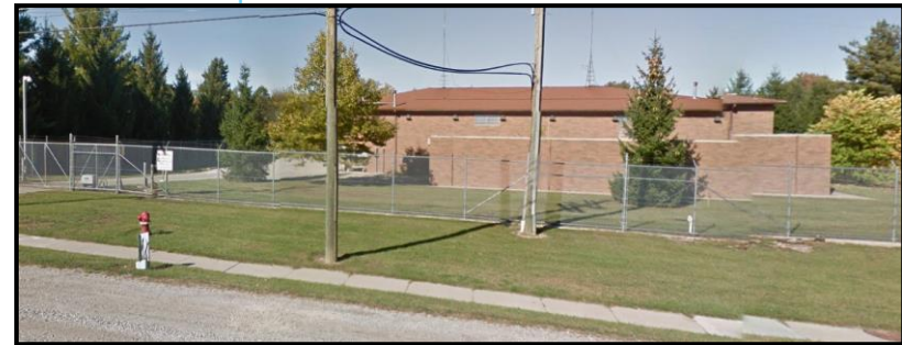
Figure 33. Rochester Pump Station
