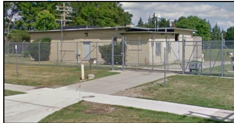
Figure 36. West Chicago Pump Station
