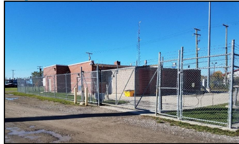
Figure 26. Michigan Avenue Pump Station
