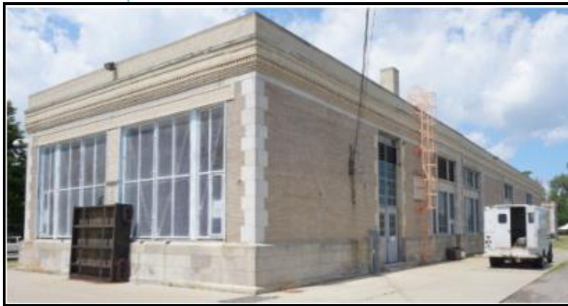
Figure 57. Fairview Pump Station
