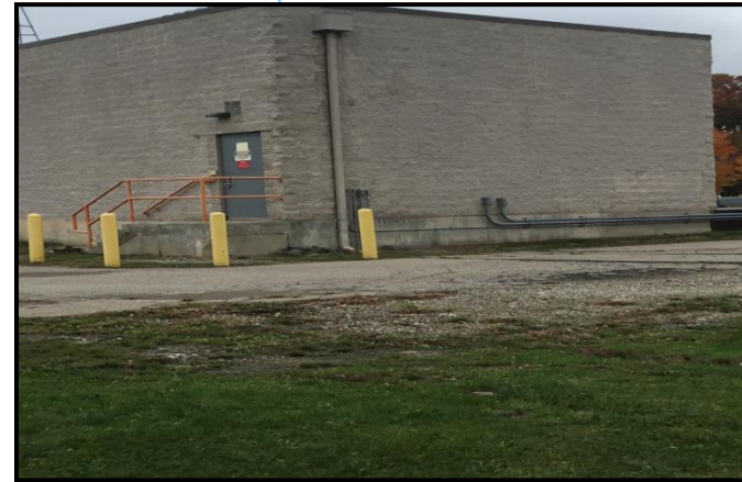
Figure 20. Adams Road Pump Station
