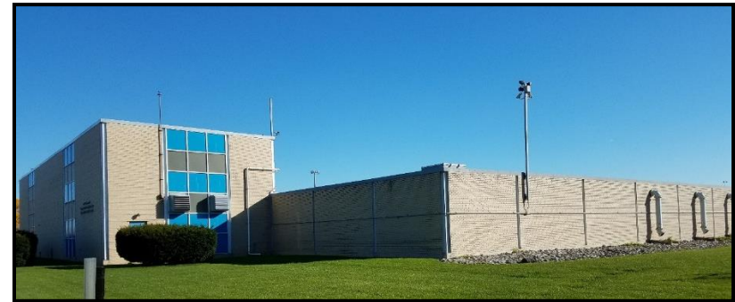
Figure 24. Ford Road Pump Station
