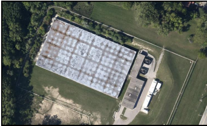
Figure 25. Franklin Pump Station
