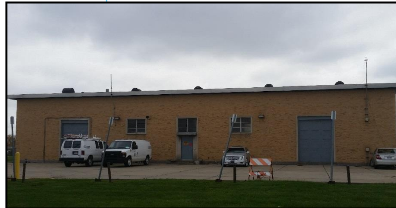
Figure 30. Northwest Pump Station
