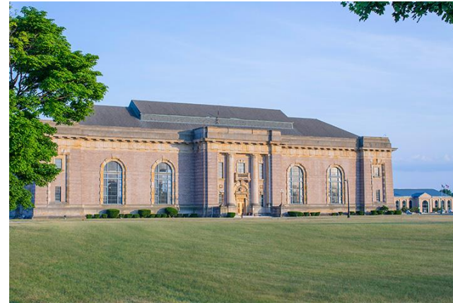
Figure 10. Water Works Park WTP
