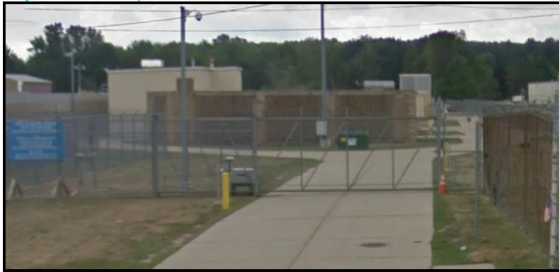
Figure 27. Joy Road Pump Station
