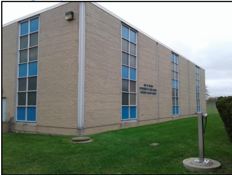
Figure 29. Newburgh Pump Station
