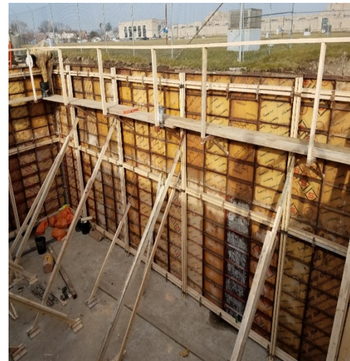
Braced Valve Vault Wall
