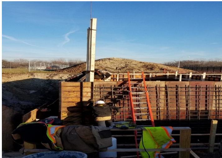
Installing bulkhead with water stop
