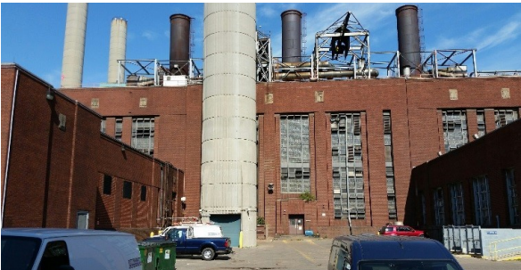
Complex – I Incinerator Building at the WRRF
