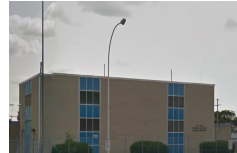
Ford Road Booster Pumping Station
