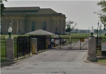
Waterworks Park WTP
