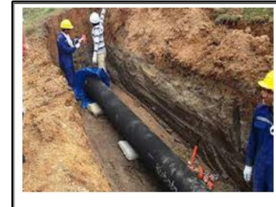
Water main being installed
