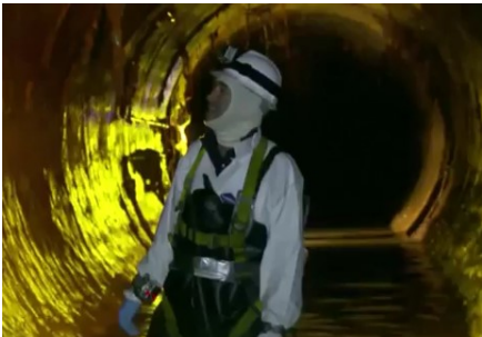
Visual inspection of a large sewer
