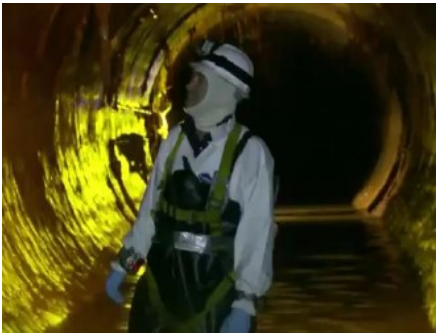
Example inspection of a large sewer
