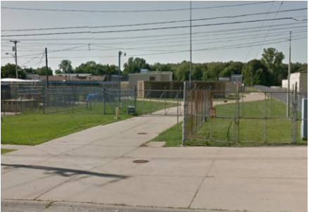
Joy Road Pumping Station
