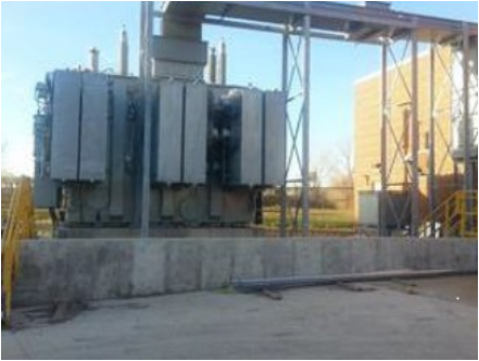
Electrical Duct Bank
