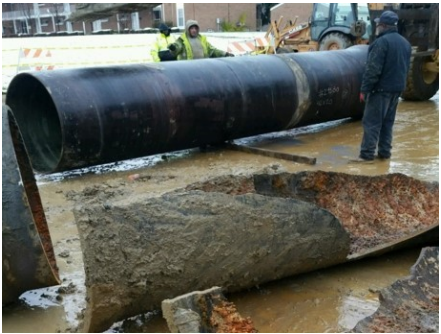
Water main replacement
