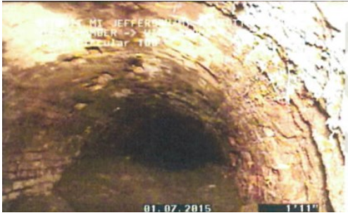
Sewer tap piping in B009 outfall (left) and sludge buildup and poor masonry in B007 outfall (right)
