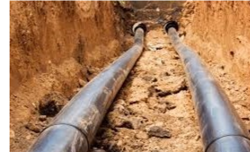
Water main installation
