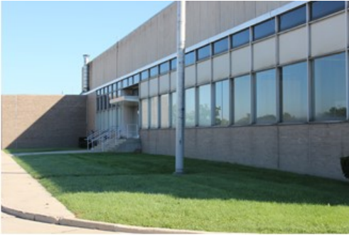
Southwest Water Treatment Plant
