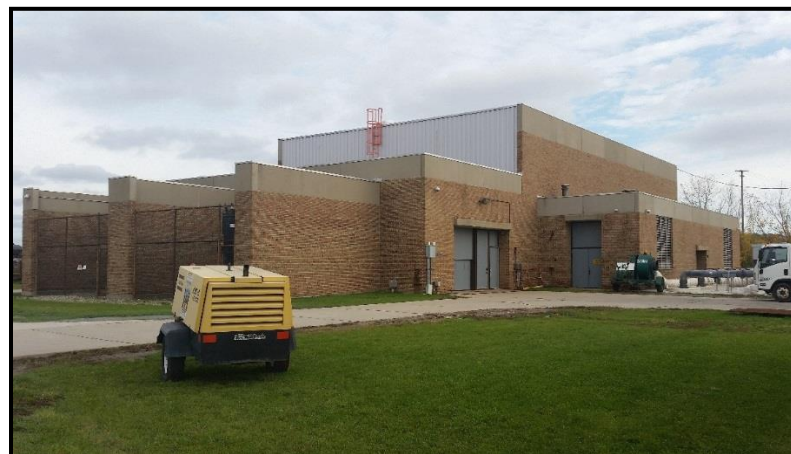
Figure VI-61. Northeast Pump Station
