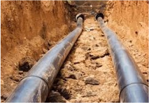
Example of pipe being laid
