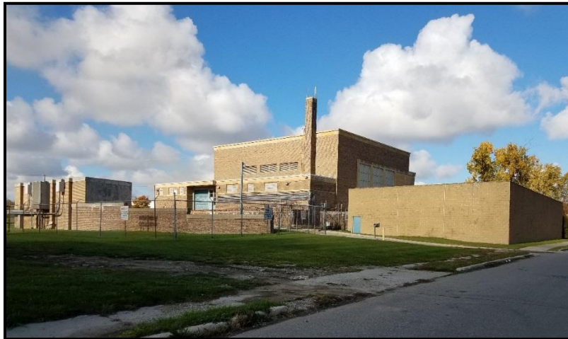
Figure VI-59. Freud Pump Station
