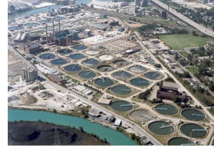
Aerial view of the WRRF
