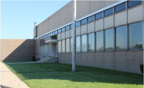
Southwest Water Treatment Plant
