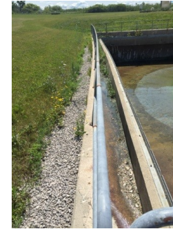
Example of concrete testing
