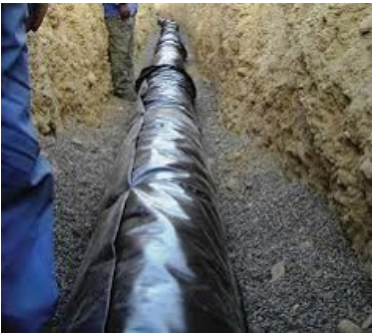
Water main being laid
