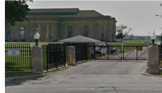
Waterworks Park WTP
