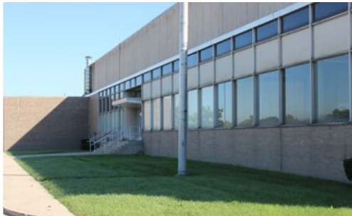
Southwest Water Treatment Plant
