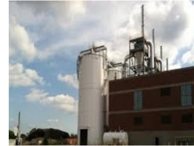
New GLWA Biosolids Dryer Facility
