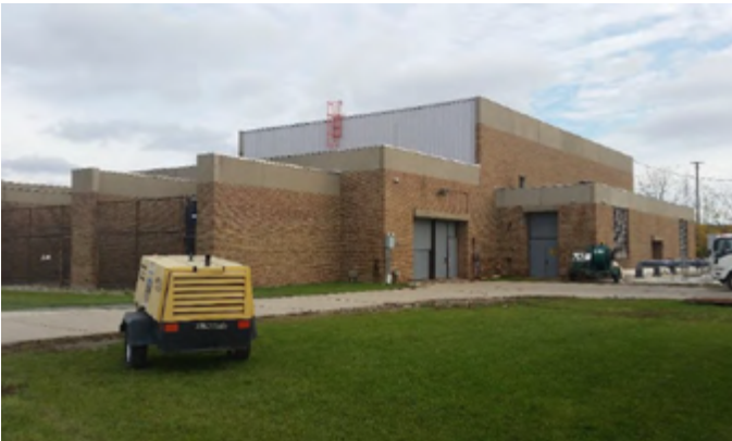
Figure 61. Northeast Pump Station
