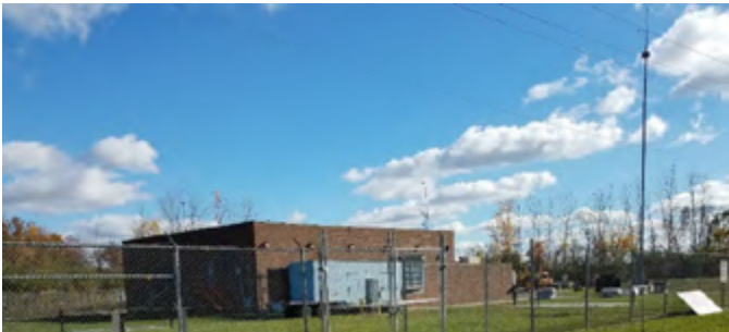
Figure 38. Ypsilanti Pump Station
