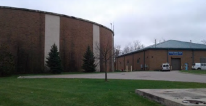
Figure 23: Haggerty Pump Station
