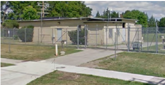
Figure 36. West Chicago Pump Station
