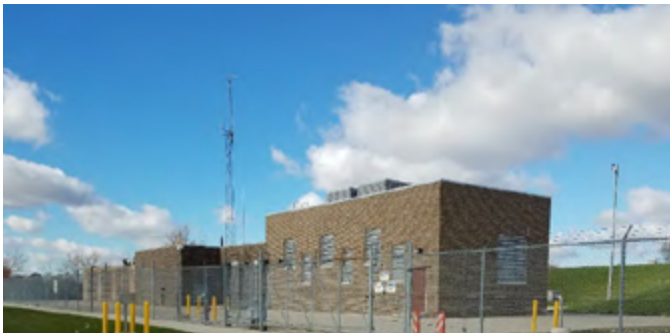
Figure 37. Wick Road Pump Station
