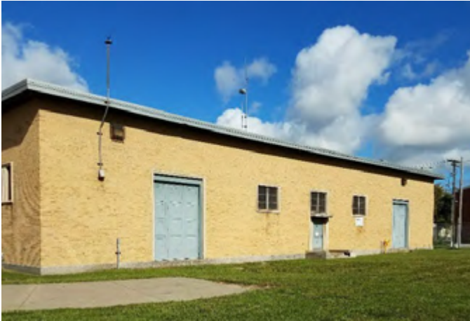
Figure 21. Eastside Pump Station
