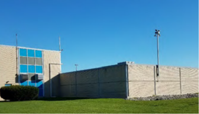
Figure 24: Ford Road Pump Station
