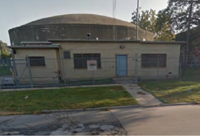
Figure 22. Electric Avenue Pump Station
