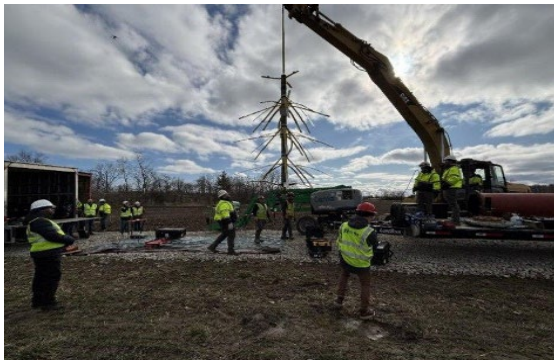
GLWA contractors preparing the PipeDiver tool for insertion into the 120" pipeline
