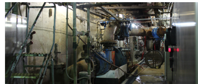
WRRF Improvements to Sludge Feed Pumps at Dewatering Facilities
