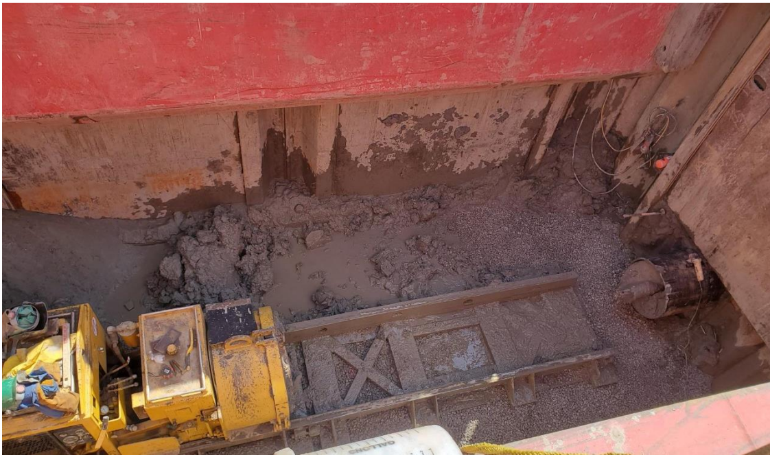
April 2023 Jacking Temporary Sludge Line Under Rail Spur
