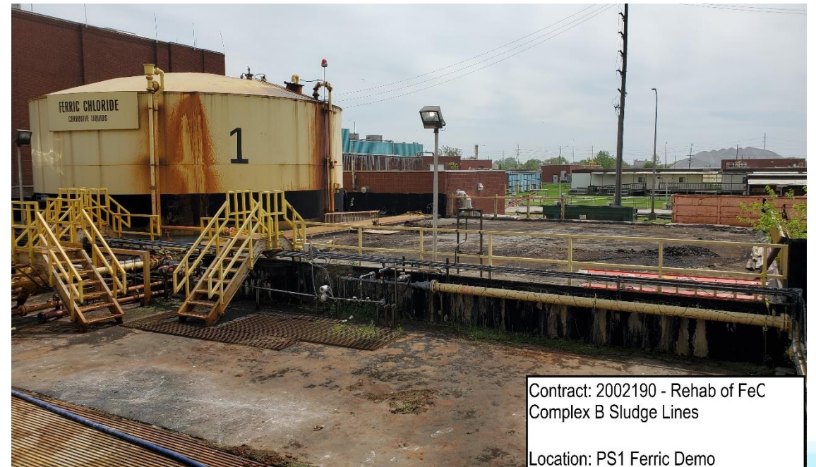
May 2023 Old Ferric Chloride Tanks Being Removed
