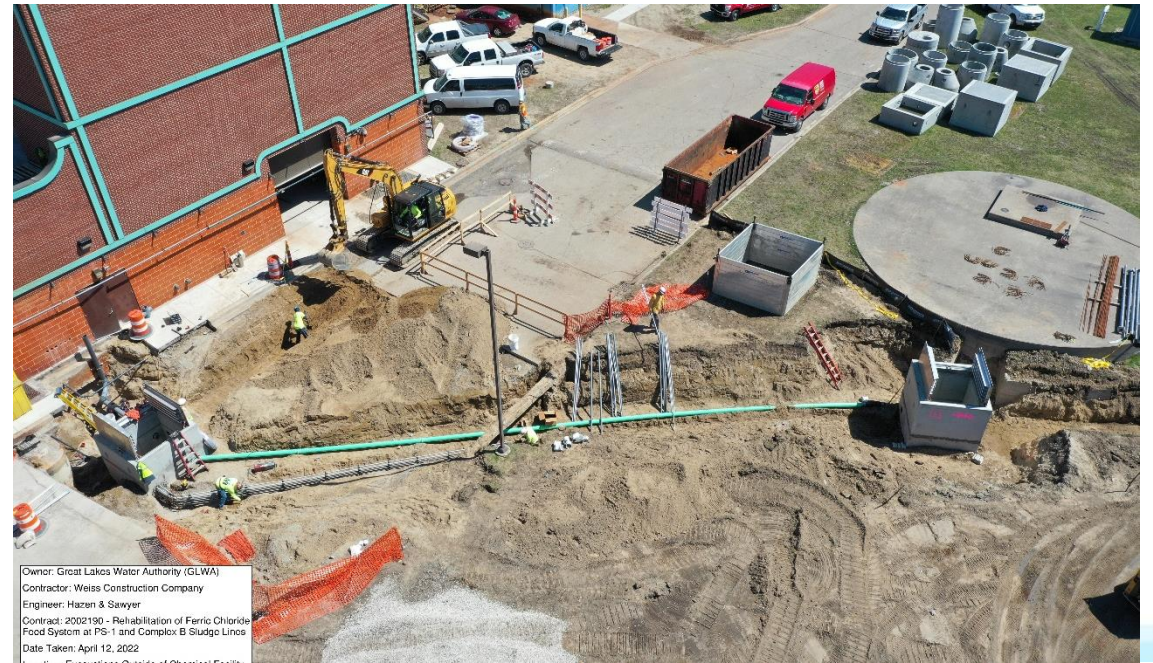
April 2022 Installing Ferric Chloride Pipeline From Chemical Building to Pump Station 1
