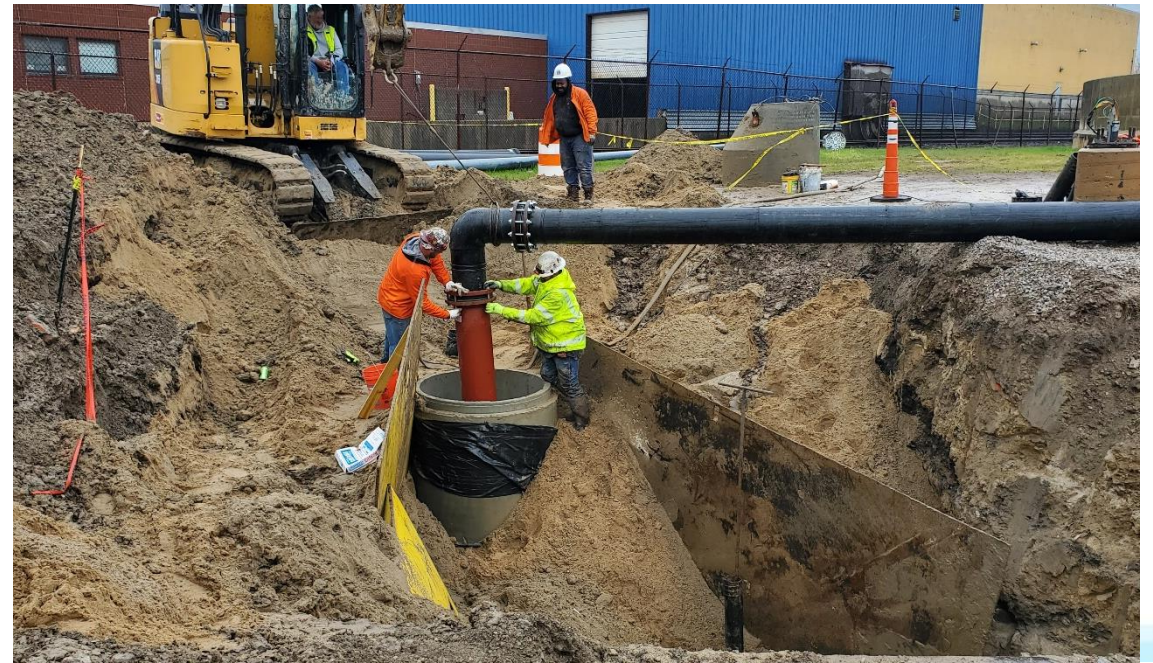
April 2023 Temporary Sludge Line Installation to Allow Chemical Cleaning
