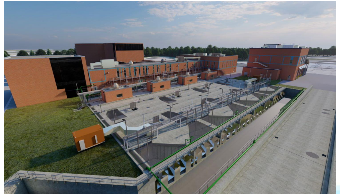
Stirred Vortex Grit Collectors (8 Total)
