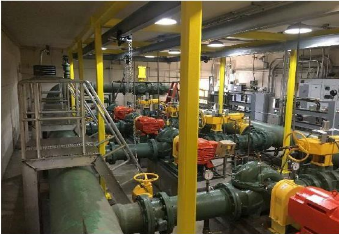
Painting of pipes and pumps
