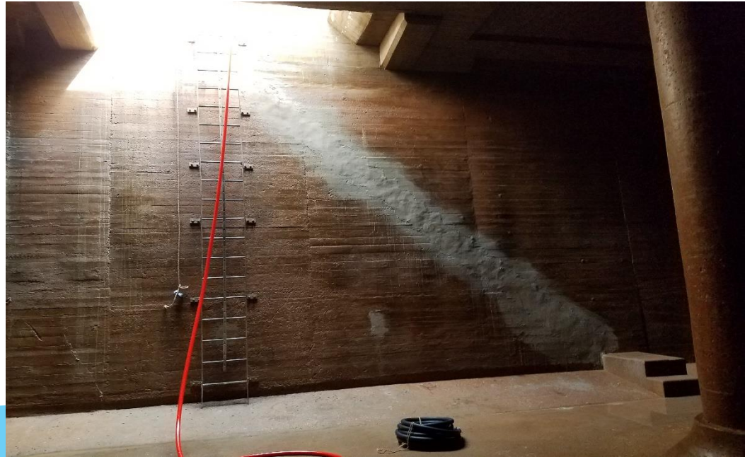
Interior Wall of Reservoir
