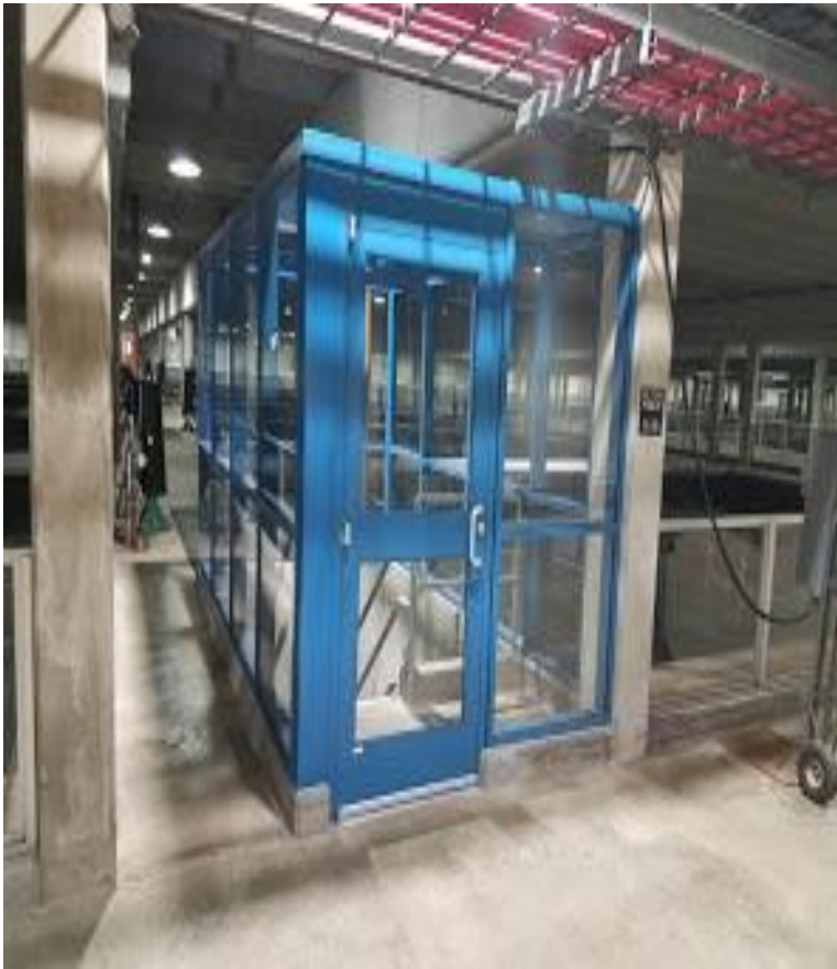
1 of 7 newly completed stairwell enclosures
