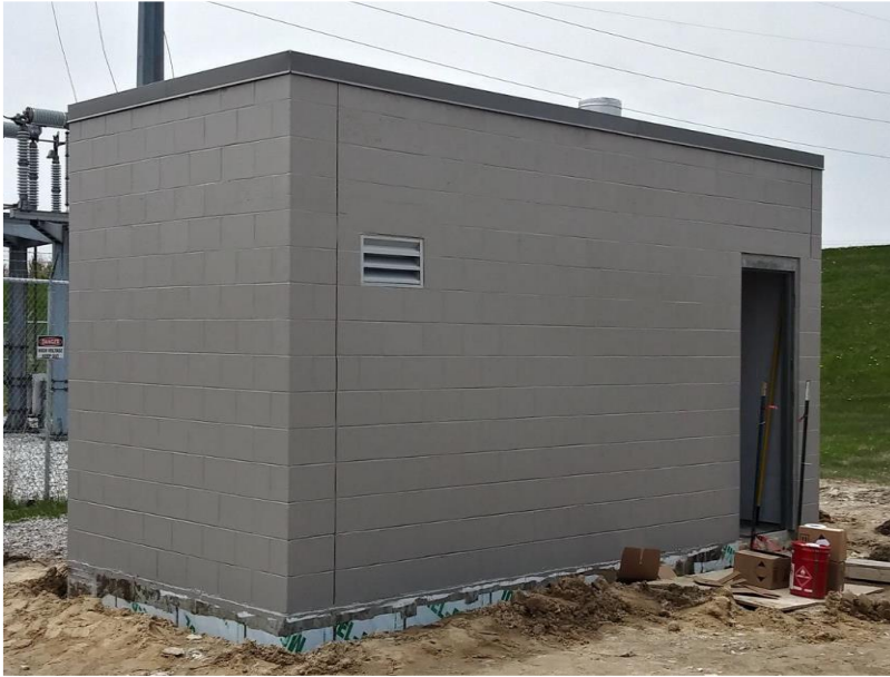
Completed exterior of stairwell structure.
