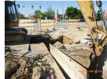
Construction on Merriman Rd.
