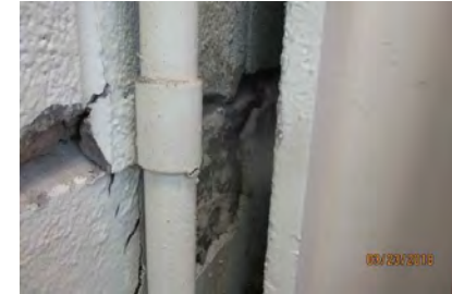
Existing Structural Condition
