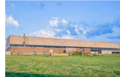
SW SCADA System Upgrade
