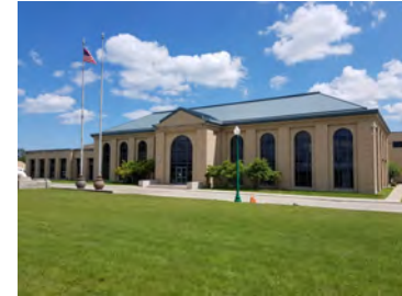
Water Works Park Water Treatment Plant
