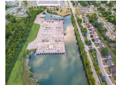
Conner Creek CSO Facility
