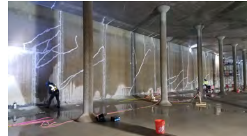
Imlay Booster Station: Sealing interior wall cracks
