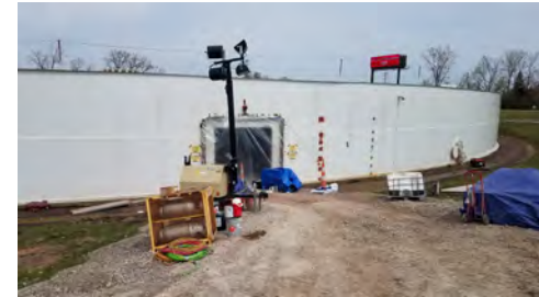
Reservoir No. 3, Access door cut into side of reservoir to perform work.
