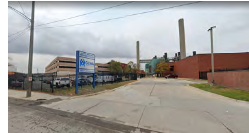
WRRF Front Entrance
