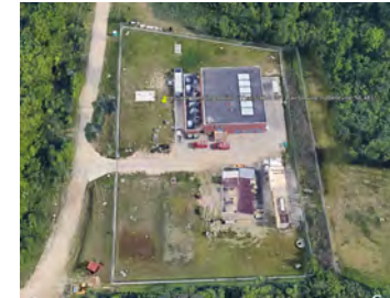
Existing Ypsi station
