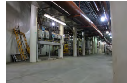
Complex B, Basement
