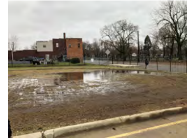
Poor Drainage at Leib
