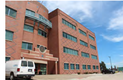
New Administration Building
