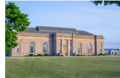
Water Works Park High Lift Pumping Station
