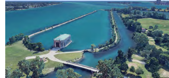
Aerial image of Belle Isle intake structure and lagoon.
