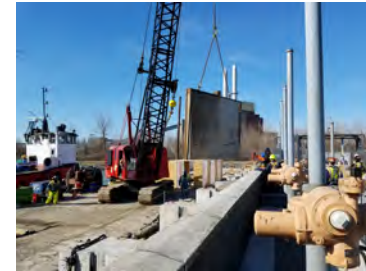
Effluent Relief Gate Repair
