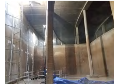
Lake Huron Plant Reservoir No. 3: Interior concrete repair.
