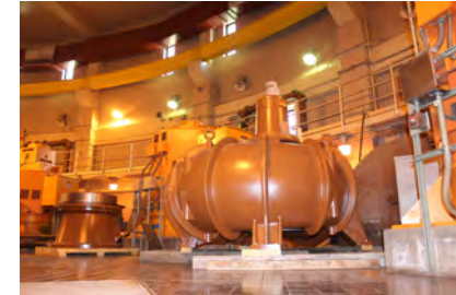
Main Raw Sewage Pumps at Pump Station 2
