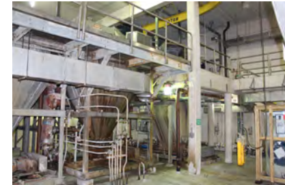
Primary Circular Scum House, Inside
