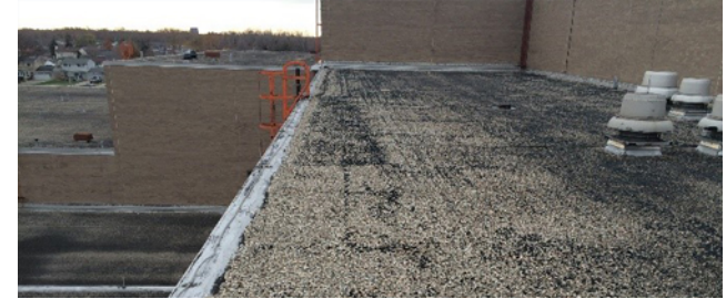
Lake Huron and Southwest Roof
