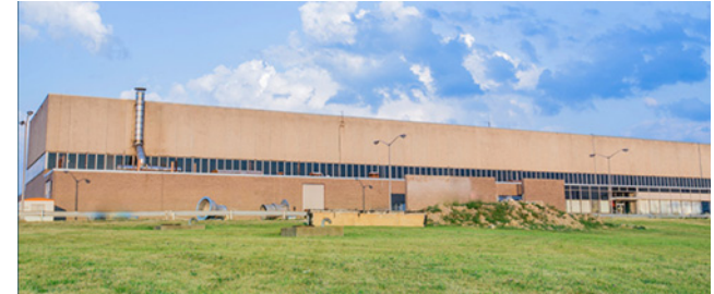
Southwest Water Treatment Plant
