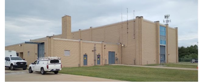
North Service Center Pumping Station
