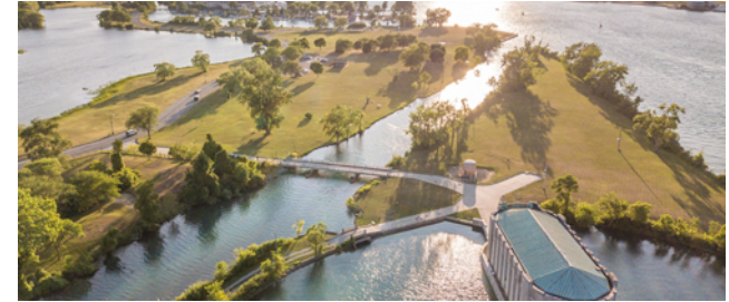
Belle Isle Intake System
