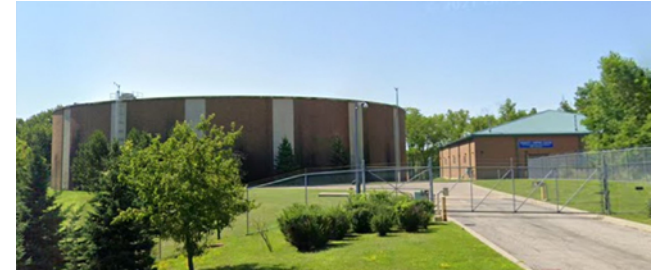
Imlay Pumping Station
