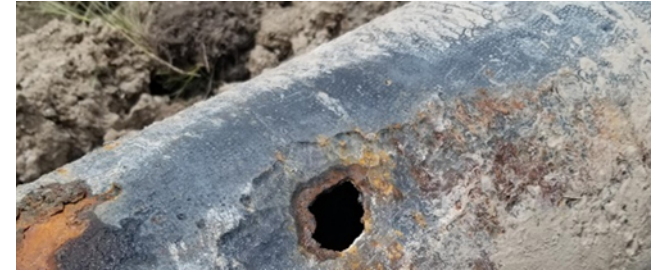
Fireloop and Plant Water Improvements
