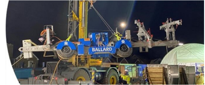
Raw Water Supply Tunnel
