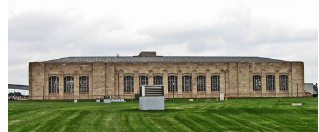
Springwells Water Treatment Plant
