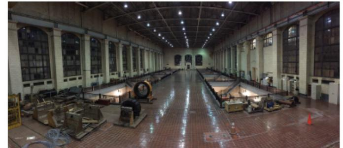
High Lift Station viewed from Low Lift Station operating floor showing high lift pump pits and windows to be replaced.
