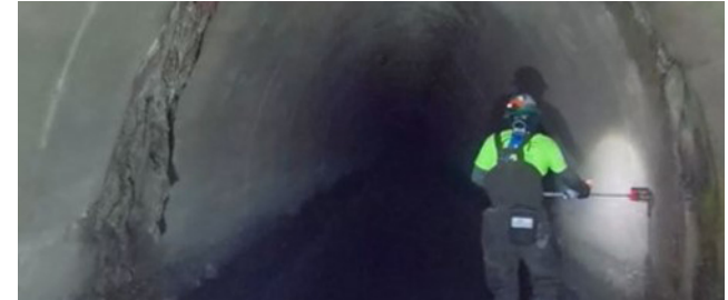
Conveyance System Repairs (Sewers)
