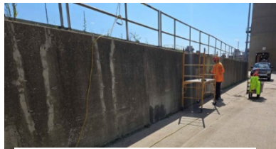
Repairs at Aeration Basin # 1
