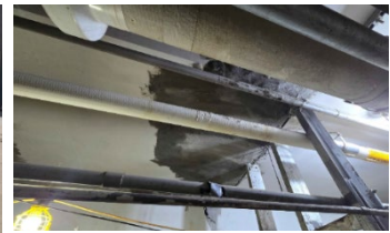
Repairs at Yard Piping tunnel
