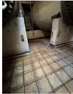
New ReSteel laid out at Venturi 3 and 4
