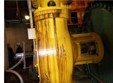
Oil hydraulic valve actuators leaking oil
