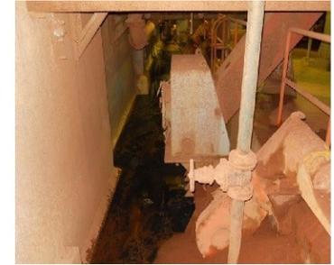
Ash crusher system was last rehabilitated 15 years ago and near the end of its useful life, due to Complex I decommissioning dry ash system needs to be reconfigured and rehabilitated
