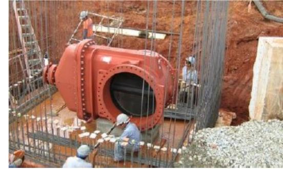
A large valve for a transmission pipe
