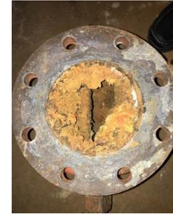
The photo shows the condition of the heating system hot water piping buildup which necessitates the complete replacement of the hot water radiant system in the filter building and other areas of the LH WTP.
