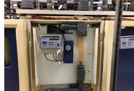
The Water Works Park Chlorine System has experienced several leaks and requires complete replacement. The Water Works Park storage room will have an updated scrubber system to neutralize up to 4000 lbs of chlorine gas
