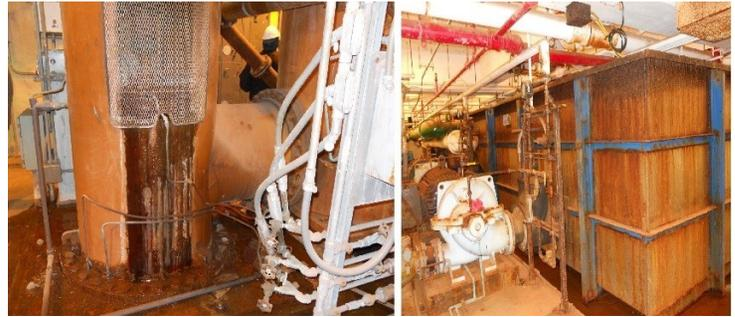
Significant SFE & Secondary Water Pump Station and pipe corrosion, requiring equipment and building rehabilitation. No redundancy for power supply to SFE pump station. Latest cooling oil test (DGA) indicates potential issues with two 5kV Transformers
