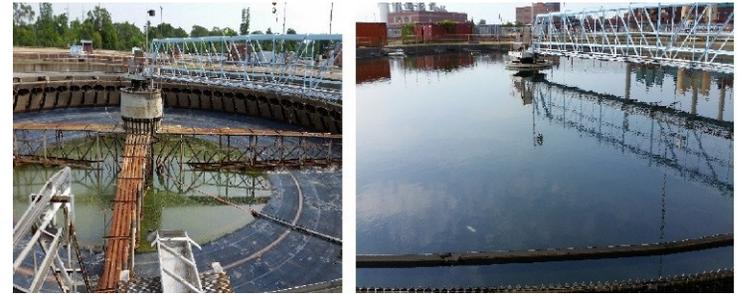
Only one or maximum two out of total 25 secondary clarifiers can be taken out of service at a time for repairs. Secondary system has a lot of moving parts and equipment. A long term (8 years) rehabilitation program for the secondary clarifiers needs to be
