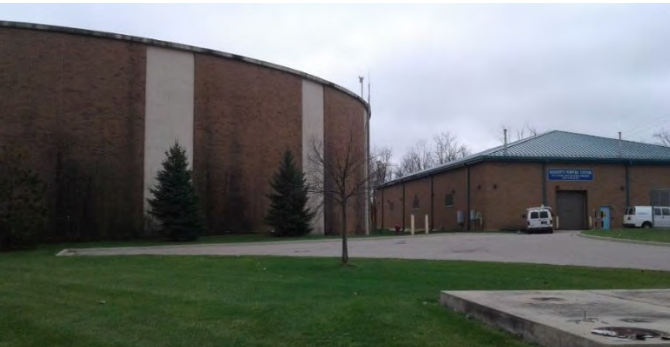
Figure 23: Haggerty Pump Station
