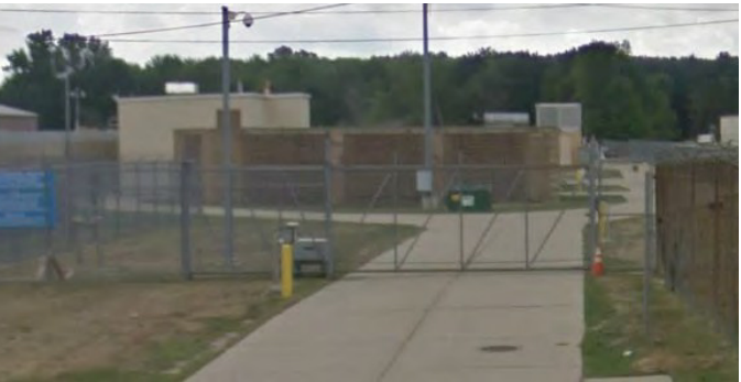
Figure 27. Joy Road Pump Station
