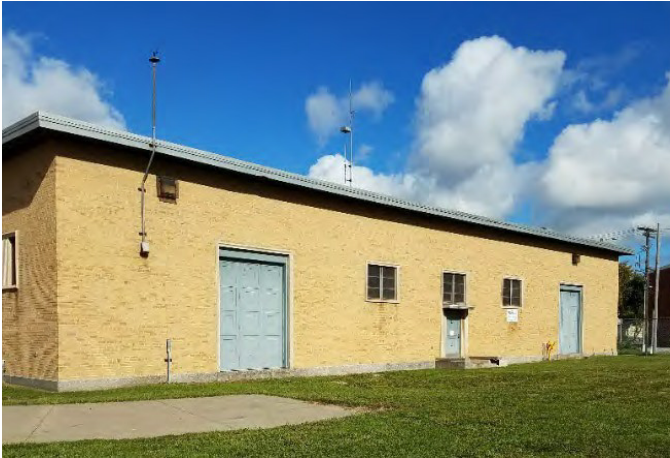
Figure 21. Eastside Pump Station
