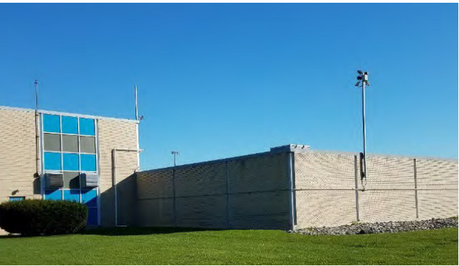
Figure 24: Ford Road Pump Station
