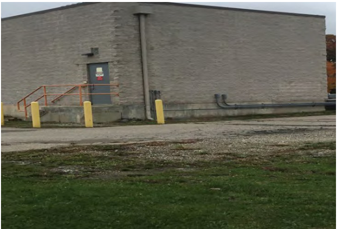
Figure 20. Adams Road Pump Station
