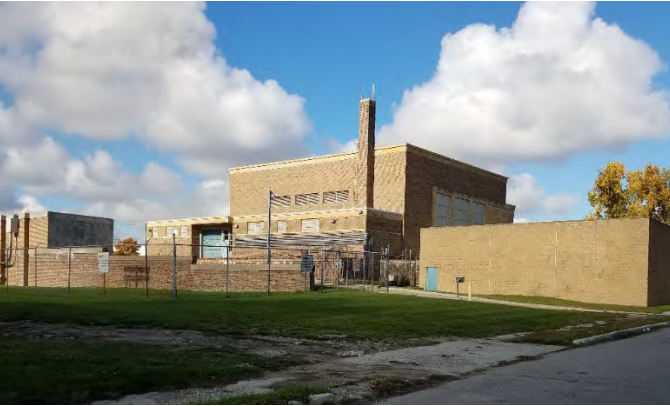
Figure 59. Freud Pump Station
