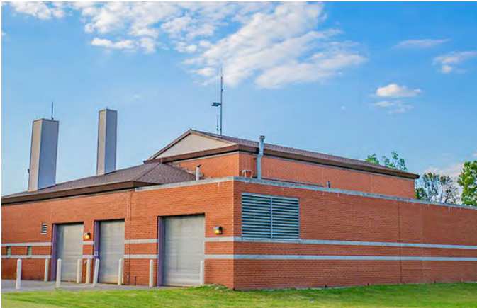
Figure 43. Puritan-Fenkell CSO RTB
