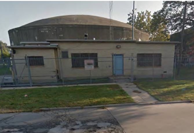
Figure 22. Electric Avenue Pump Station
