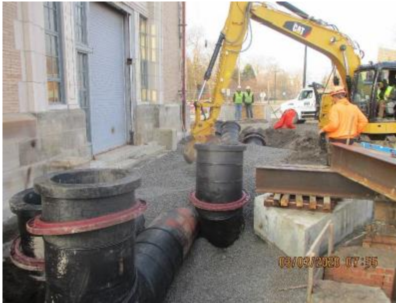
Trench Backfilling with gravel
