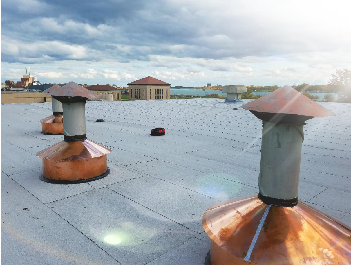
Water Works Park Raw Water Booster Station – New Roofing and Vent Flashing
