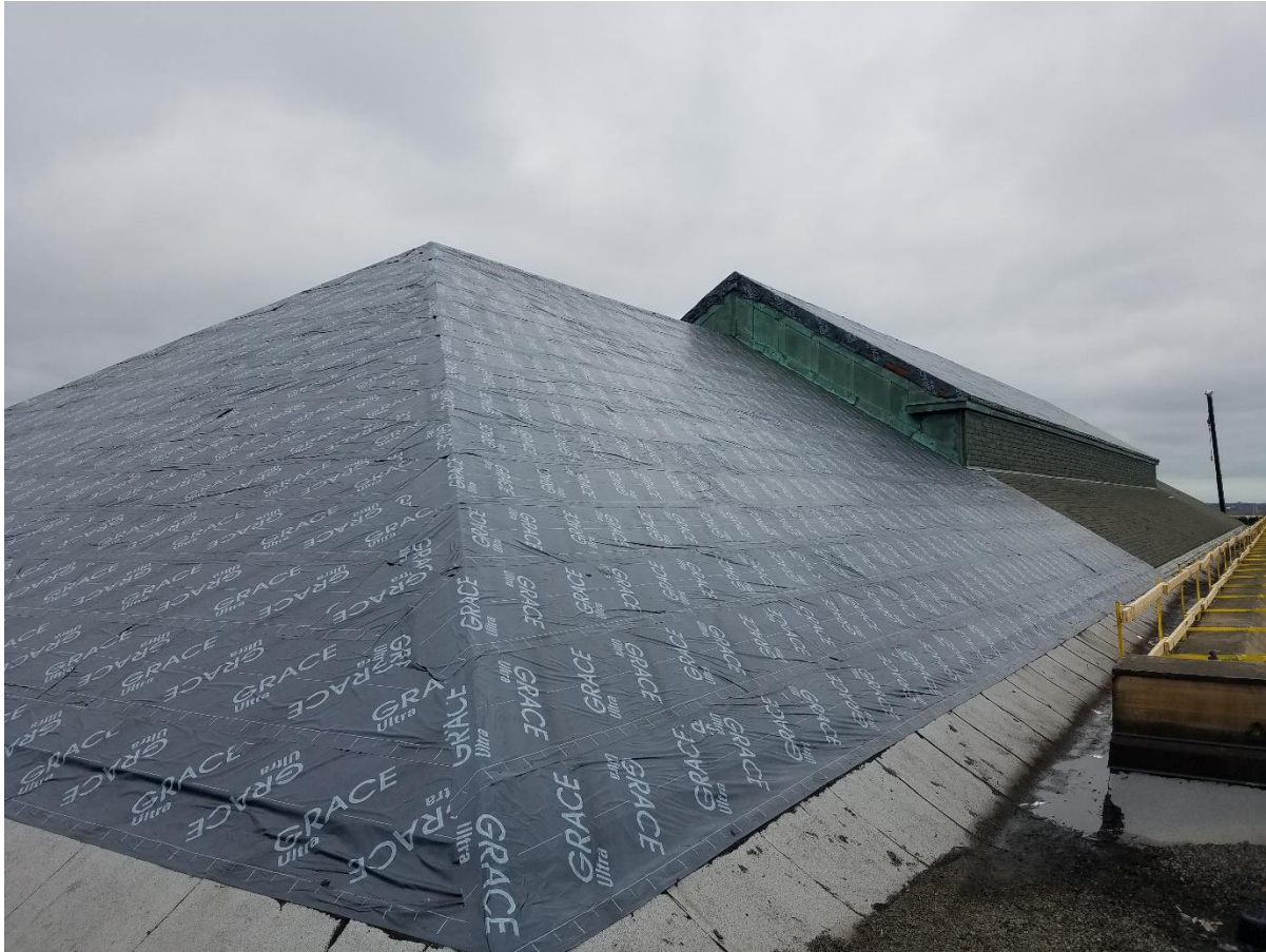
WWP High-Lift Building – Installation of Ice & Water Shield
