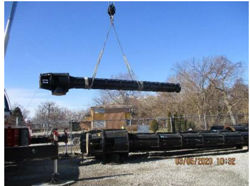
Lifting of Pumps
