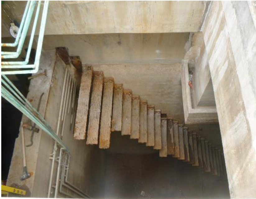
Demo of Staircase Basin #1 (2020)
