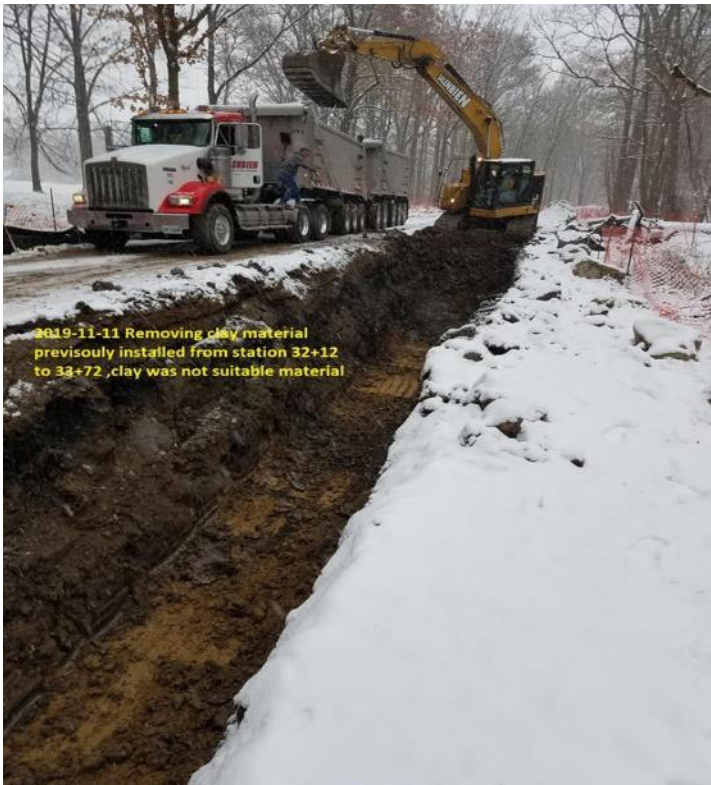
Excavation for 24-Inch Transmission Main
