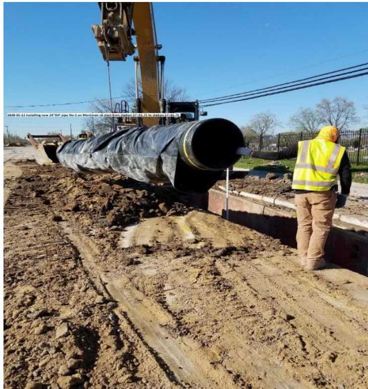
Installation of 24-Inch Transmission Main
