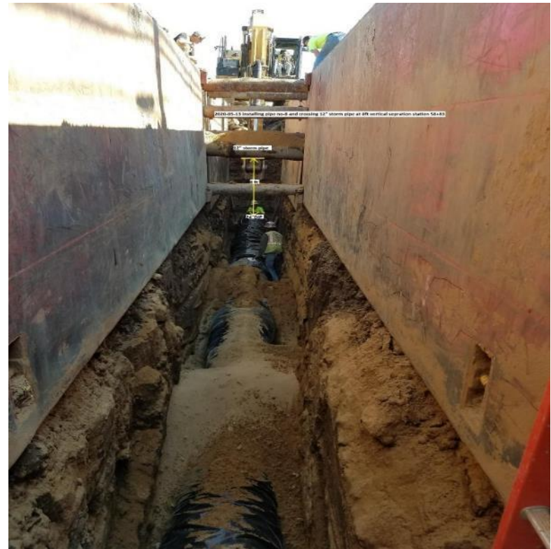
Backfill of 24-Inch Transmission Main
