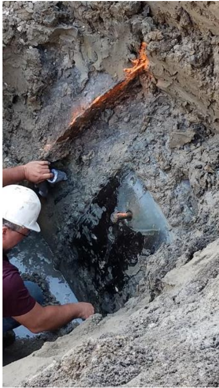
Main #5 Leak Repair
