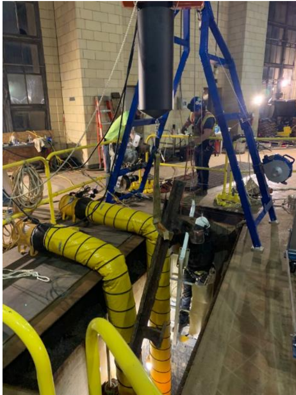
Removal of Gate Guides
