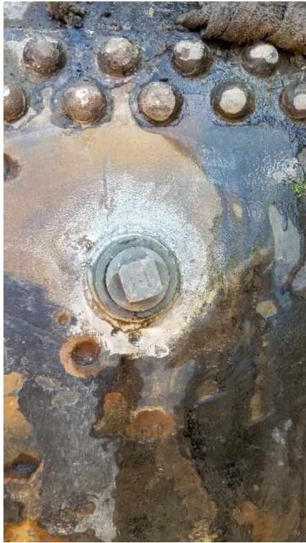
Repaired Riveted Steel Pipe
