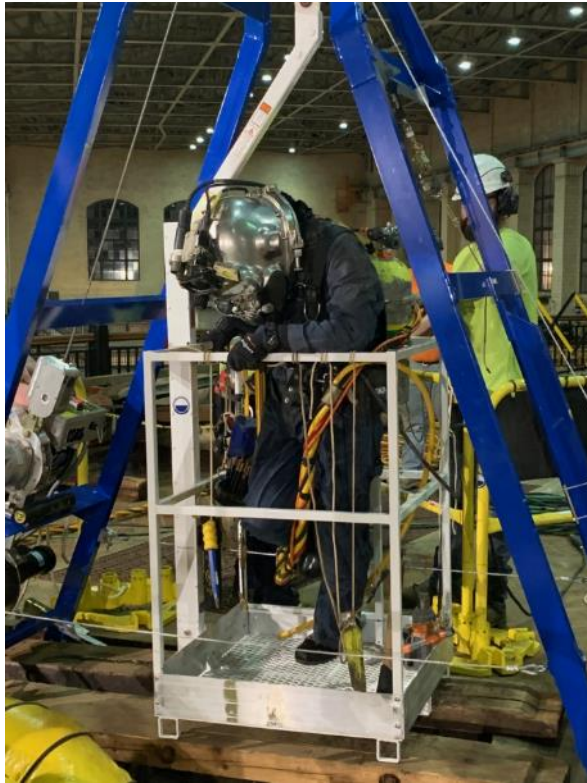
Diver Preparing for Entry
