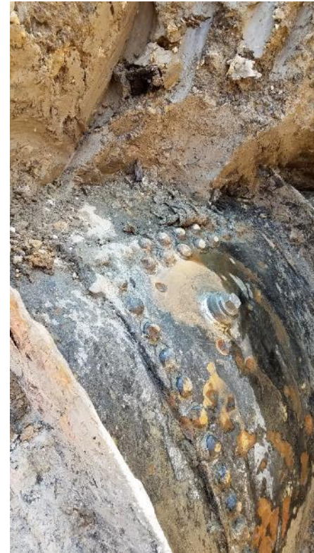
Main #5 Leak Repair
