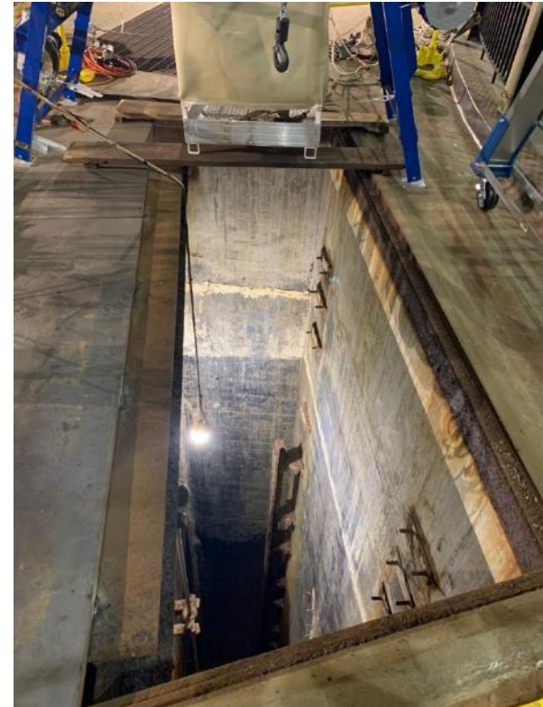
View of Suction Well
