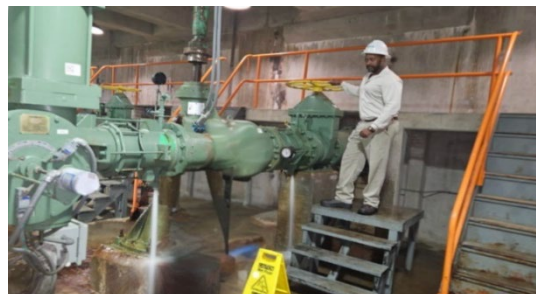
Justin Woods at the Northwest Pumping Station attempting to isolate control valve #3
