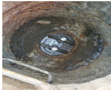
Leaking access hatch at Nevada Avenue and Fenelon Street
