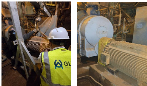
Vacuum pump A motor is being reinstalled under Team Leader Richard Muntz's guidance - shown in the left photo and the fully reassembled vacuum pump A is shown in the right photo.
