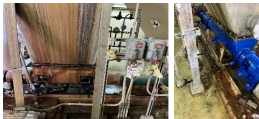
The old scum hopper grinder is shown in the left photo and the new model installed is shown in the right photo.
