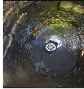
Gratiot Road and Seven Mile Road, 8-inch gate leak
