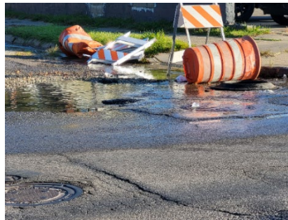
Leaking access hatch at Nevada Avenue and Fenelon Street
