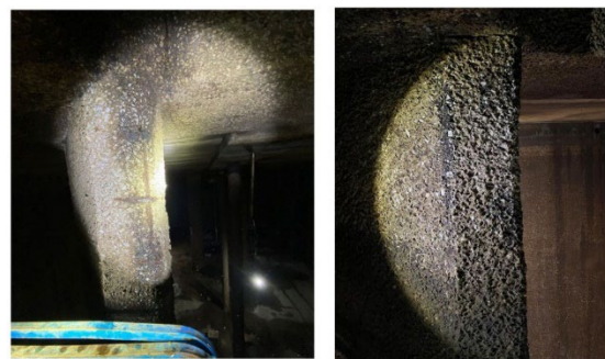
Aeration Deck 2 Mixer column deterioration.
