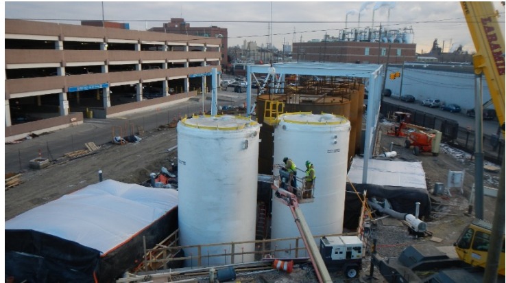
Hypo building construction in progress
