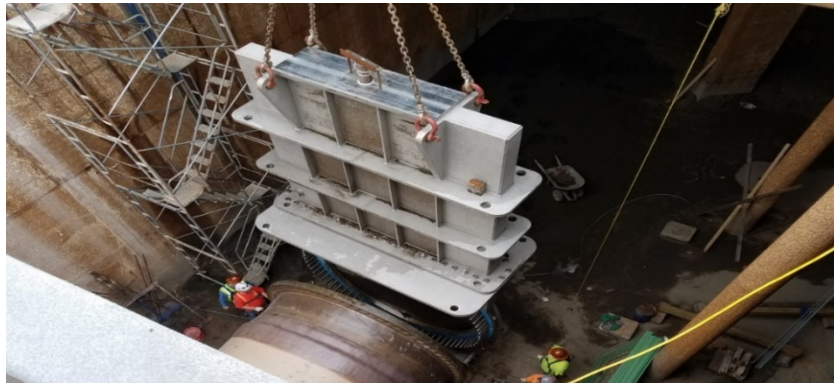
120-inch diameter Knife Gate valve installation in Aeration Basin No. 2
