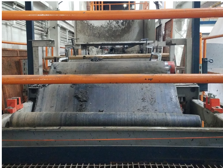
Complex II Incineration N Belt repair in process
