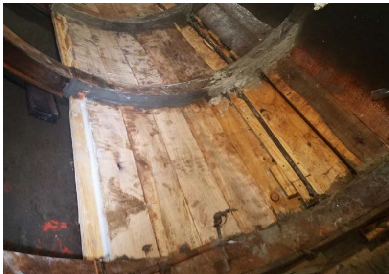
Lagging Installation between Ribs
