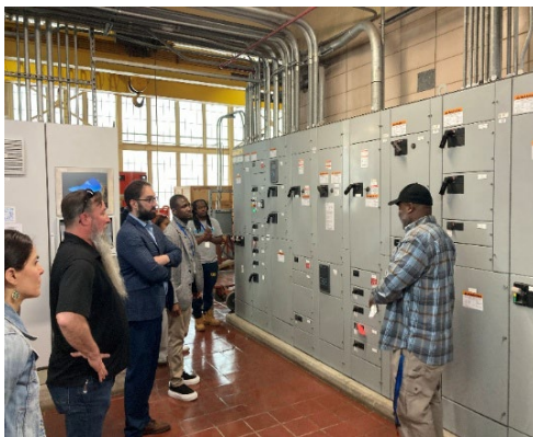
GLWA Team Leader Darvin Fox explains the pump start-up process at the Baby Creek CSO Facility on April 22 nd .
