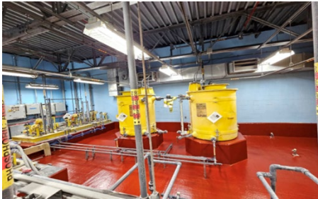
After: Containment area
