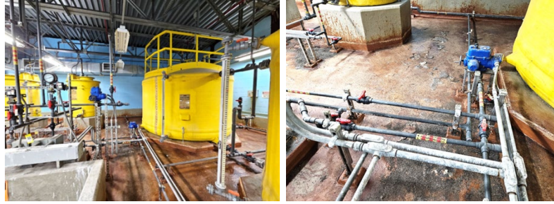
Before: containment area
