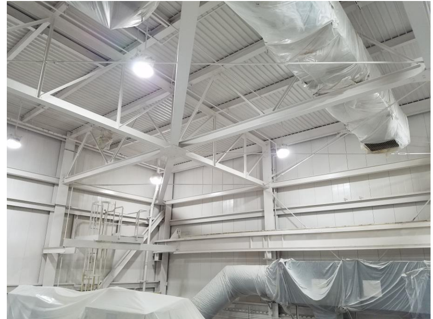
Dewatering II Repainting
