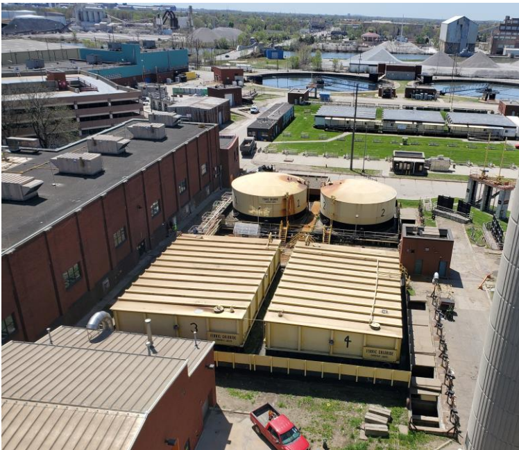
Existing ferric chloride storage tanks will be demolished at PS-1 grit tank process area
