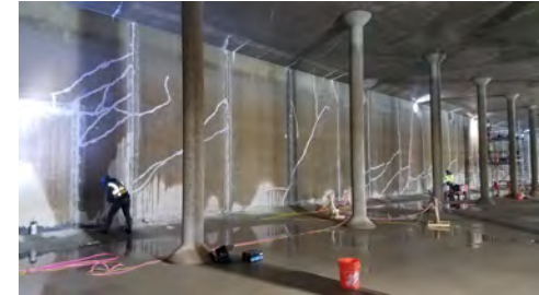
Imlay Booster Station: Sealing interior wall cracks
