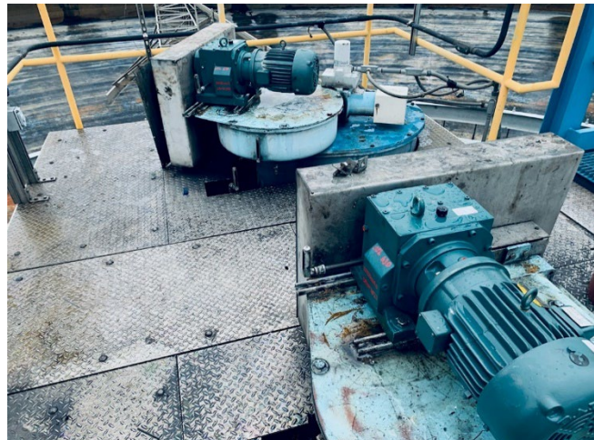
New motors and gearboxes installed on primary clarifier 13.
