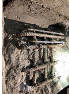
Conner Creek corbel repair
