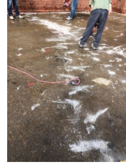
Baby Creek crack injection
