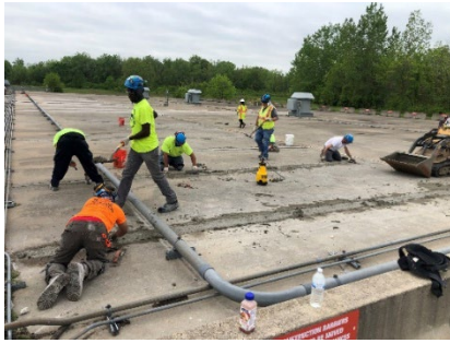
Joint repairs at Hubbell-Southfield
