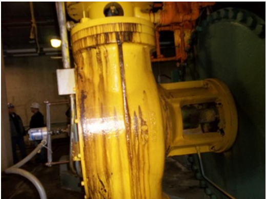
Oil hydraulic valve actuators leaking oil
