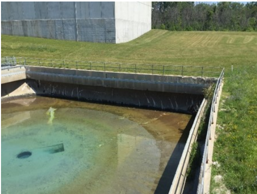
Raw sludge clarifier at Lake Huron WTP
