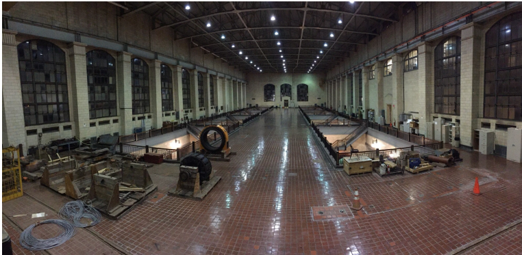
High Lift Station viewed from Low Lift Station operating floor showing high lift pump pits and windows to be replaced.
