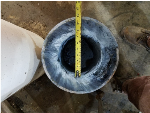
Complex B Sludge Lines clogged due to Struvite
