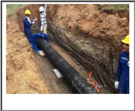
Water main being installed
