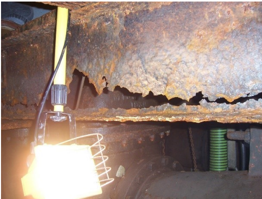
Deteriorated support beams holding up Low Lift Station. Dewatering and Sump Pumps at Elev. 42’-0” (left). Deteriorated grating and access ship’s ladder in Low Lift Station - Looking down at Elev. 50’-0” and 42’-0” from Elev. 62’-0” (right).
