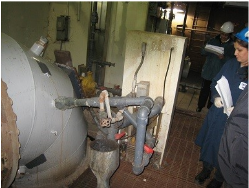
The RAS-3 sampling station in the basement of Intermediate Lift Pump No. 2 (ILP No. 2) Building samples the return activated sludge flows to Aeration Deck No.4
