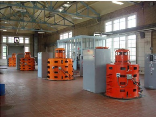
Sanitary pumps at Fairview Pumping Station
