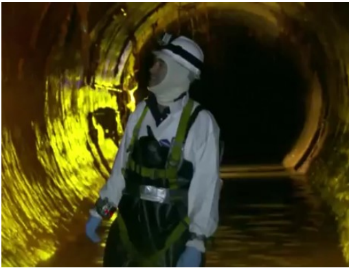
Visual inspection of a large sewer
