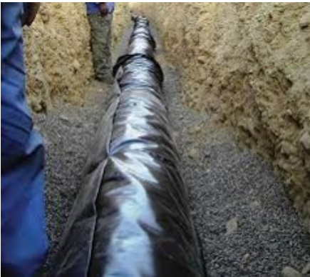
Water main being laid
