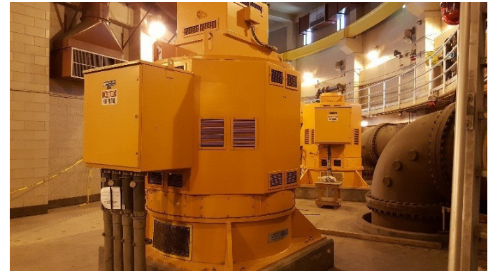
Main Raw Sewage Pumps at Pump Station 2
