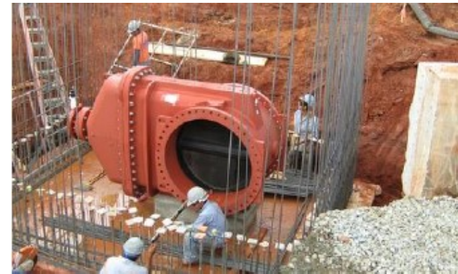
A large valve for a transmission pipe
