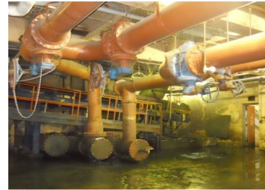
Sludge Feed Pumps
